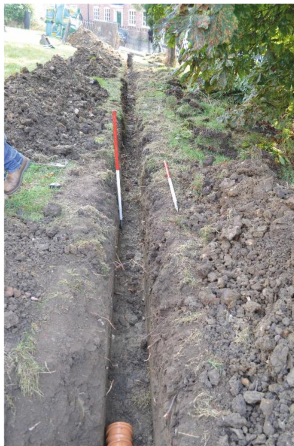
Pl. 28 Pipe trench run looking south-west towards Bolton Lane
