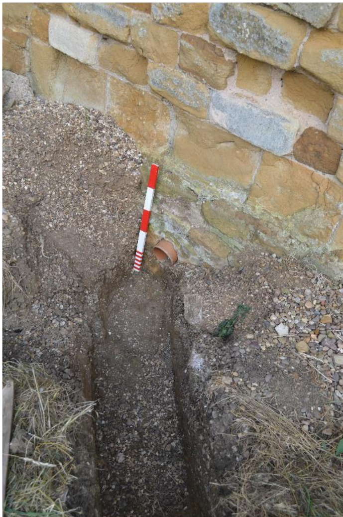
Pl. 25 Junction of pipe trench and south aisle. Scale 0.50m
