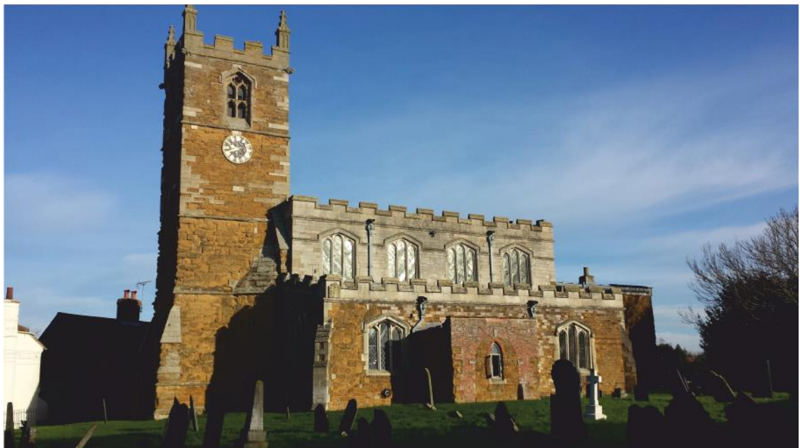
Pl. 2 Hose St Michael and All Angels church south elevation, showing south porch
