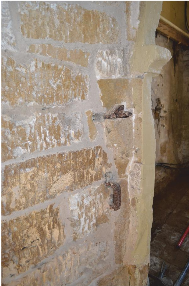
Pl. 5 South aisle door eastjamb showing door latch, looking south
