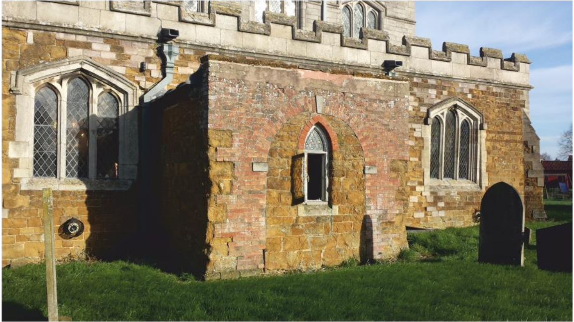
Pl. 3 The south porch showing blocked entrance with brick repairs and inserted window
