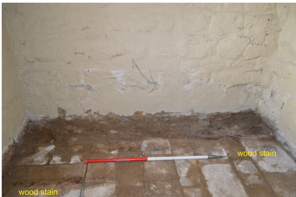
Pl. 10 South porch interior showing area of the bench position against the west wall and stains of battens on the flagstones for a timber floor predating the concrete floor, looking west. Scale 1m
