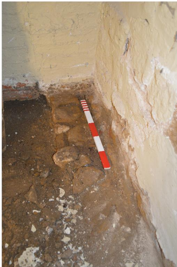
Pl. 12 Porch west wall foundations, looking south. Scale 0.50m
