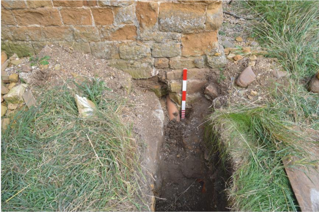
Pl. 23 Junction of pipe trench with porch west wall. Scale 0.50m
