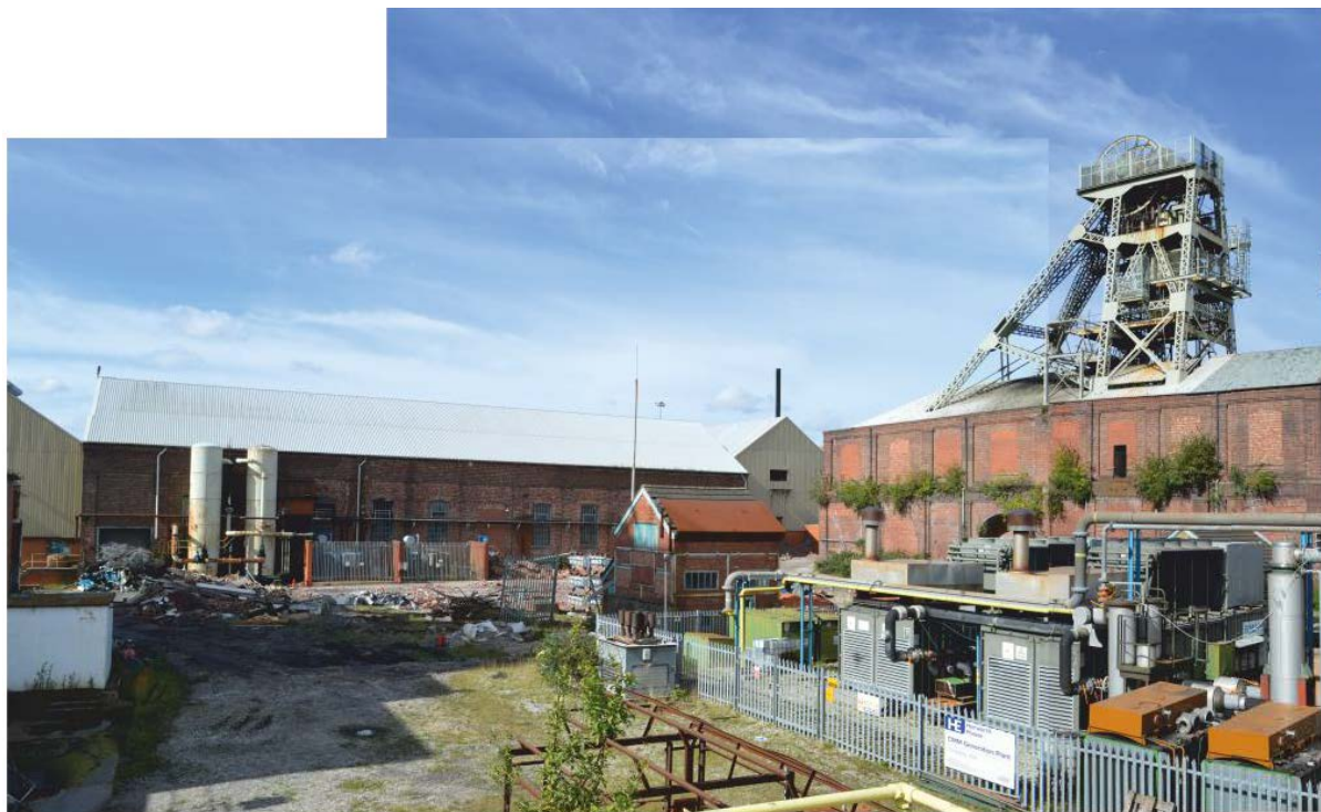
Pl. 15 Main power house and pit head no. 1 looking north-west.
