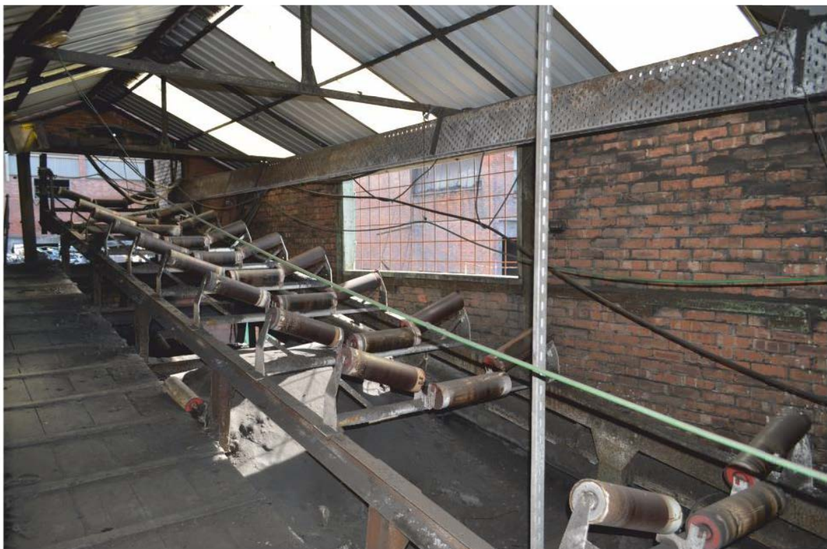
Pl.20 Conveyor belt from No. 2 shaft leading to the ROM stock tower
