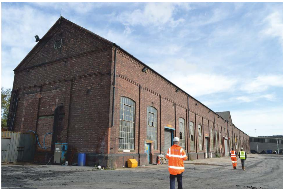
Pl. 11 Main workshops, looking east (to be retained)
