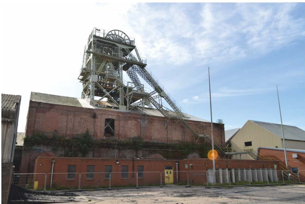
Pl. 12 Pit shaft no. 1, looking south (to be retained)
