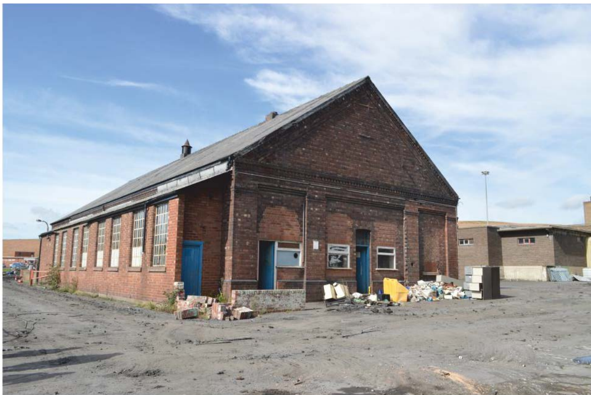
Pl. 13 Rescue room and cycle shed, looking north-west
