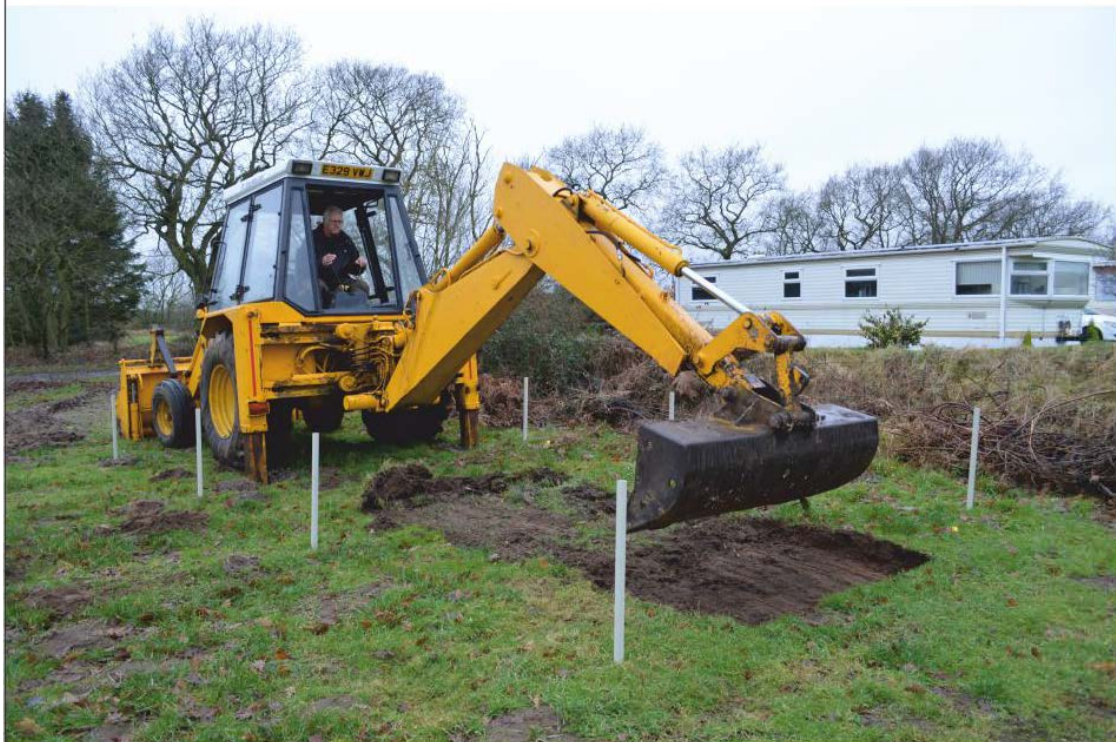
Plate 1: General view of area of Trenches 1&2, looking north
