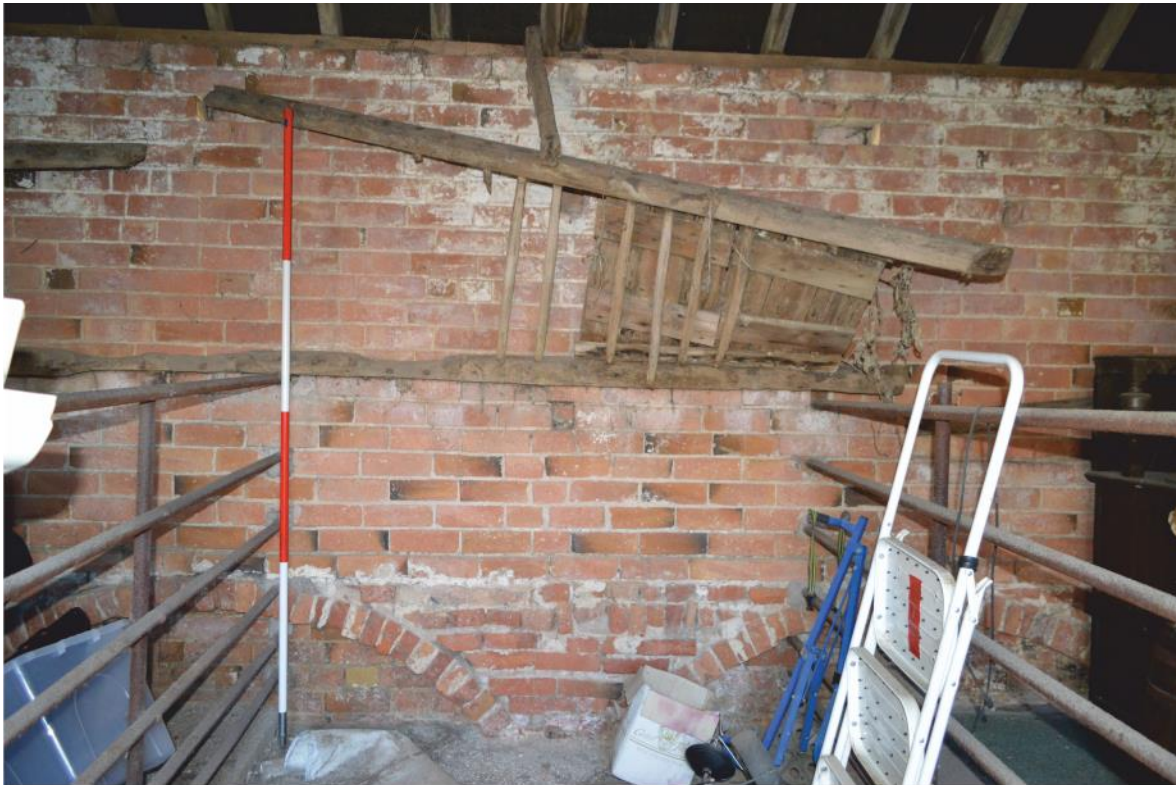
Pl. 37 Building 5, hay rack on north-west wall
