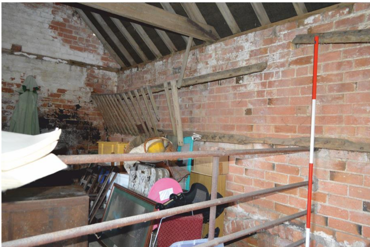
Pl.38 Building 5, hay rack on north-west wall
