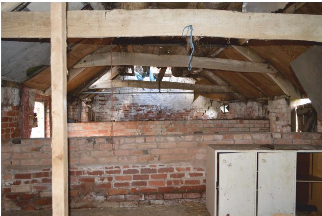
Pl. 26 Building 3 looking south-east
