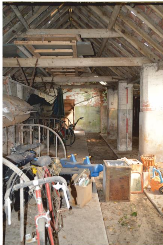
Pl. 60 Building 9, looking north-east, note the polygonal brick pillars for the cart shed
