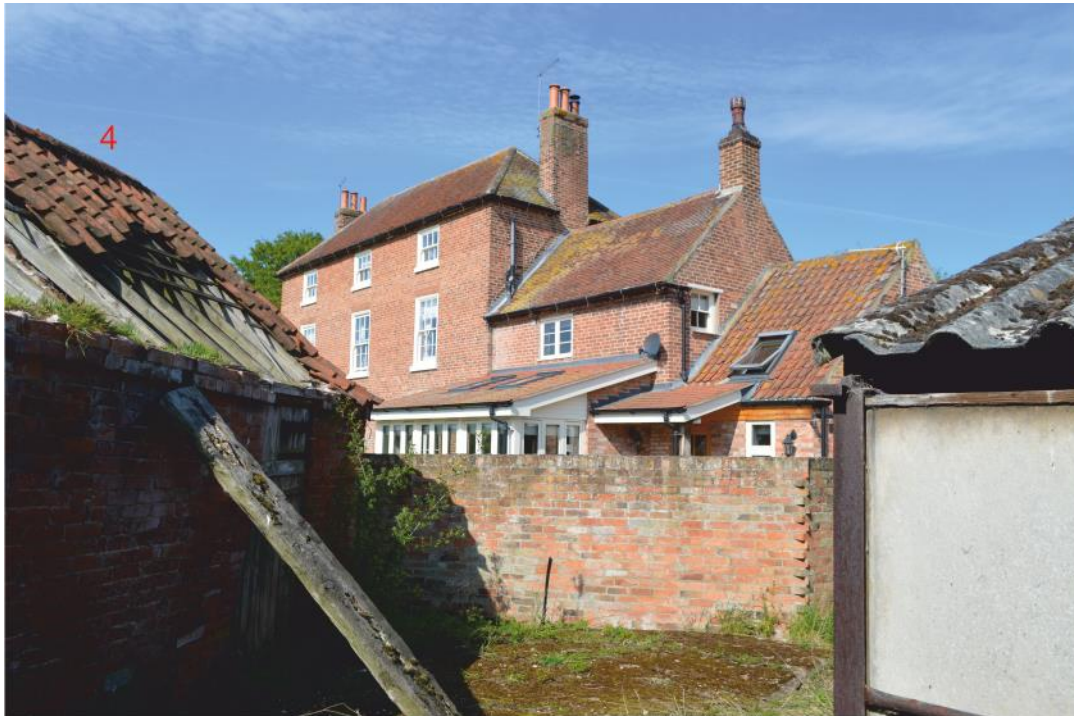
Pl. 5 Gibsmere House and building 4, looking south-west.
