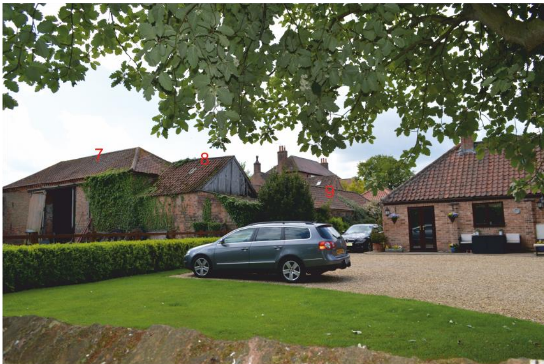
Pl 2 General view of the site looking south showing buildings 7,8,9
