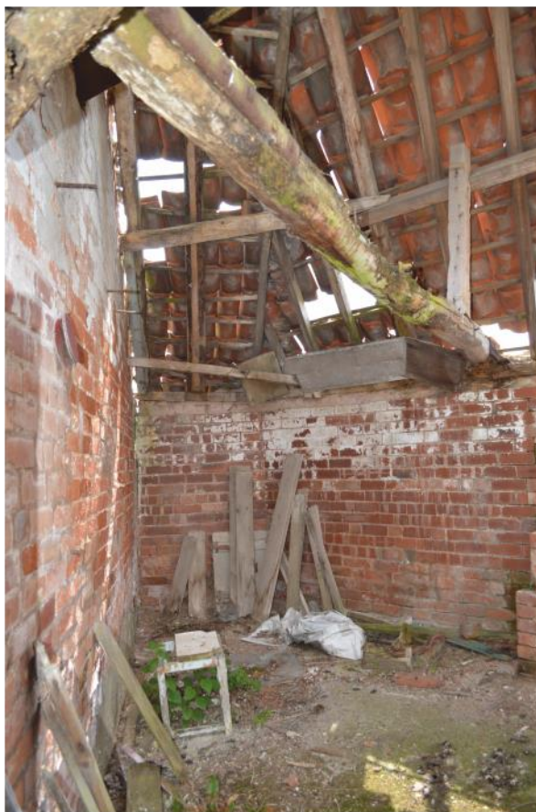
Pl. 32 Building 4a interior
