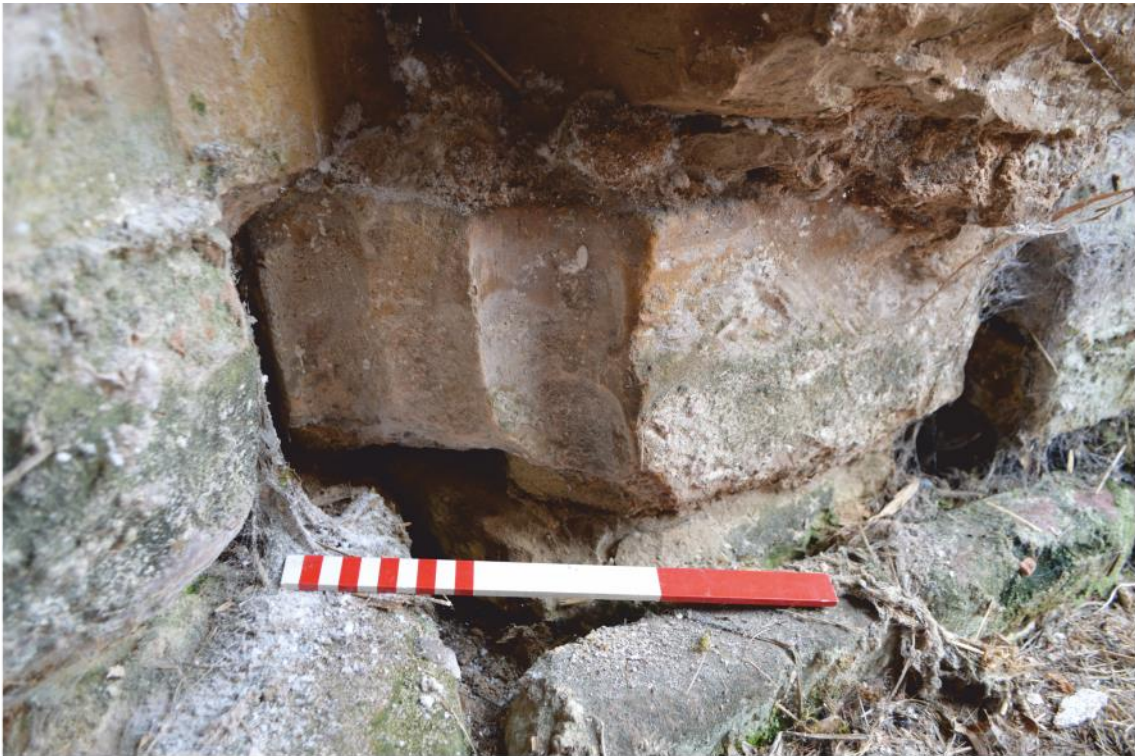
Pl. 17 Architectural fragment reused in stone plinth at base of wall
