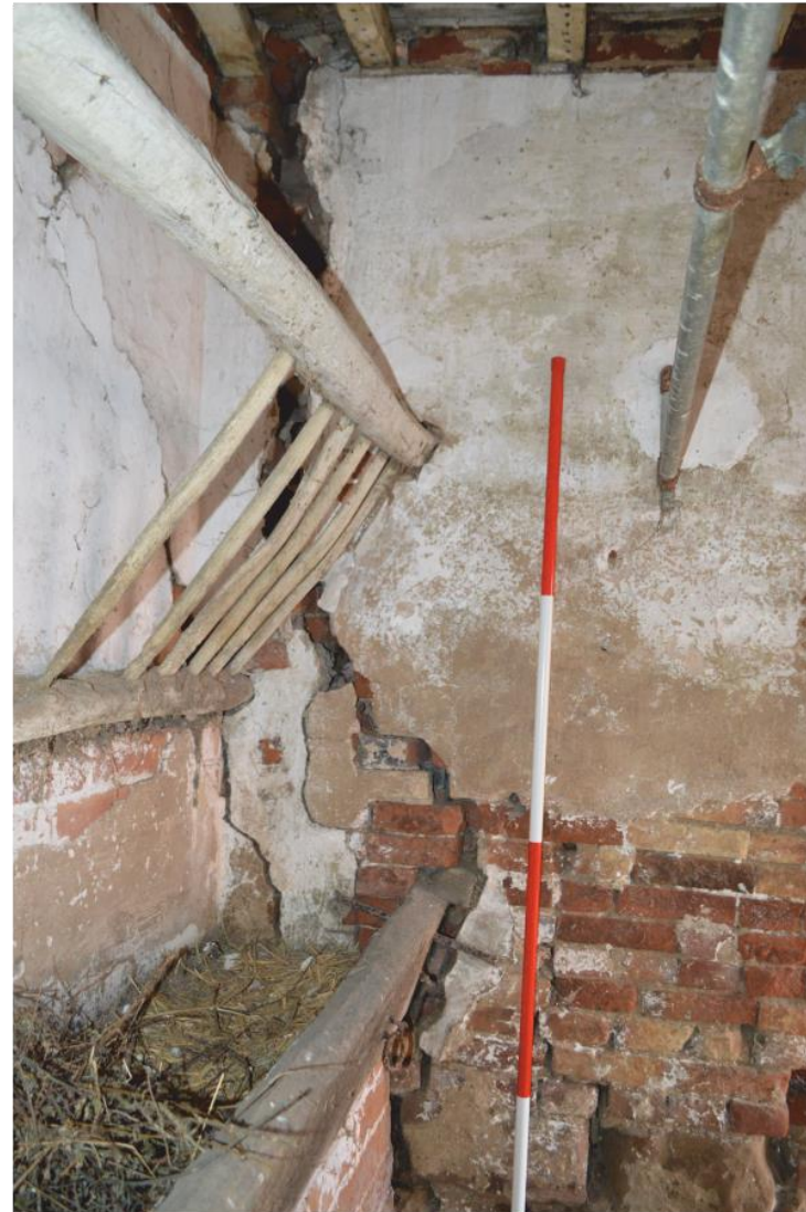
Pl. 16 Building 1b detail of inserted hay rack and feeding trough
