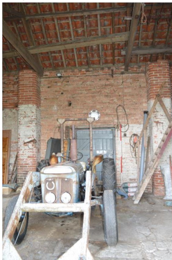
Pl. 48 Building 7, threshing barn, blocked door with inserted entrance internal elevation
