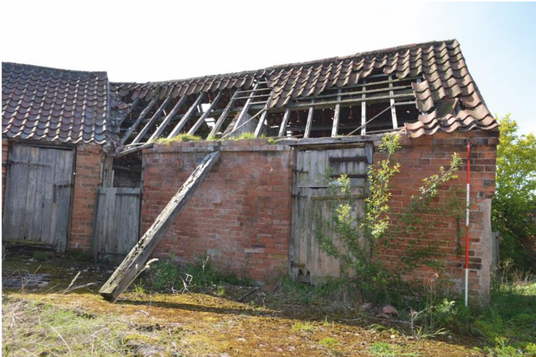
Pl. 31 Building 4 north elevation
