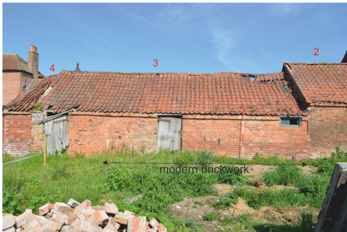
Pl. 22 Building 3 viewed from the field, much rebuilt with inserted window
