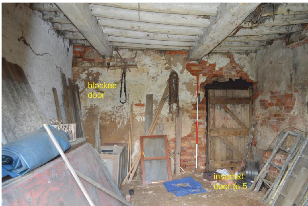
Pl. 12 Building 1a interior showing blocked door, and inserted door to building 5
