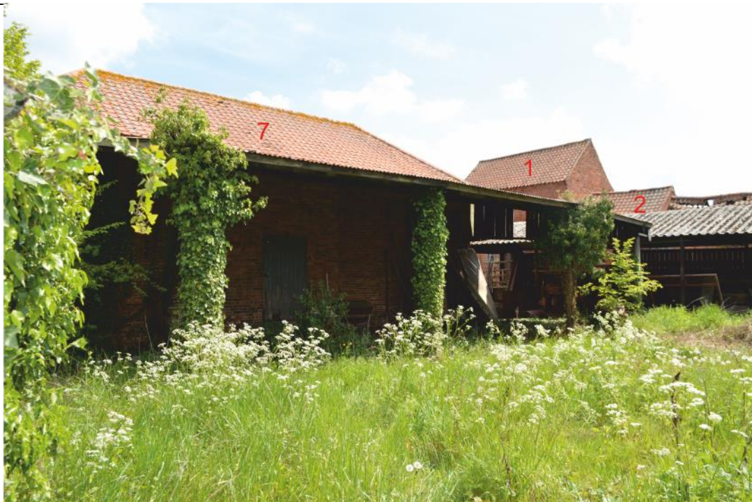
Pl. 7 General view of site looking north-east, from inside the crewyard showing buildings 7, and 1 to rear
