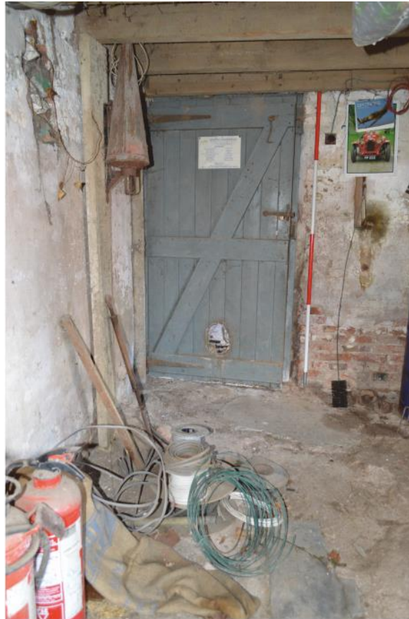
Pl. 51 Inserted door in threshing barn 7 into building 8
