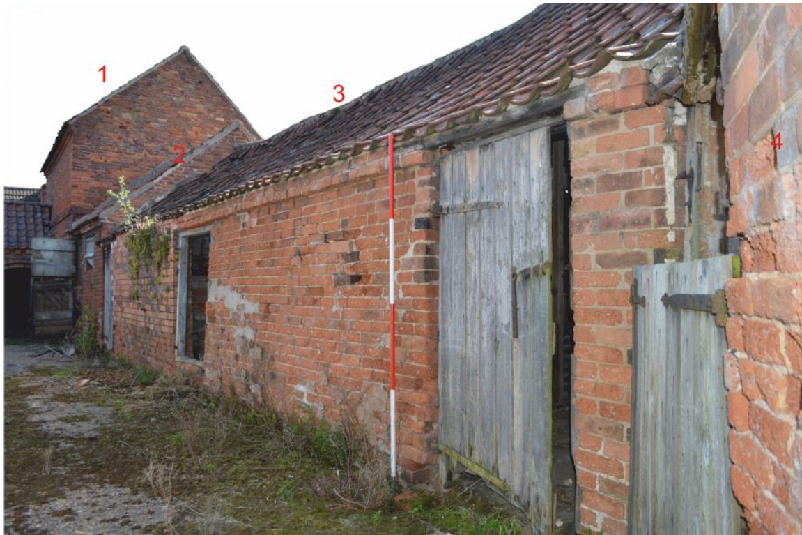
Pl. 23 Building 3 external elevation facing the crewyard
