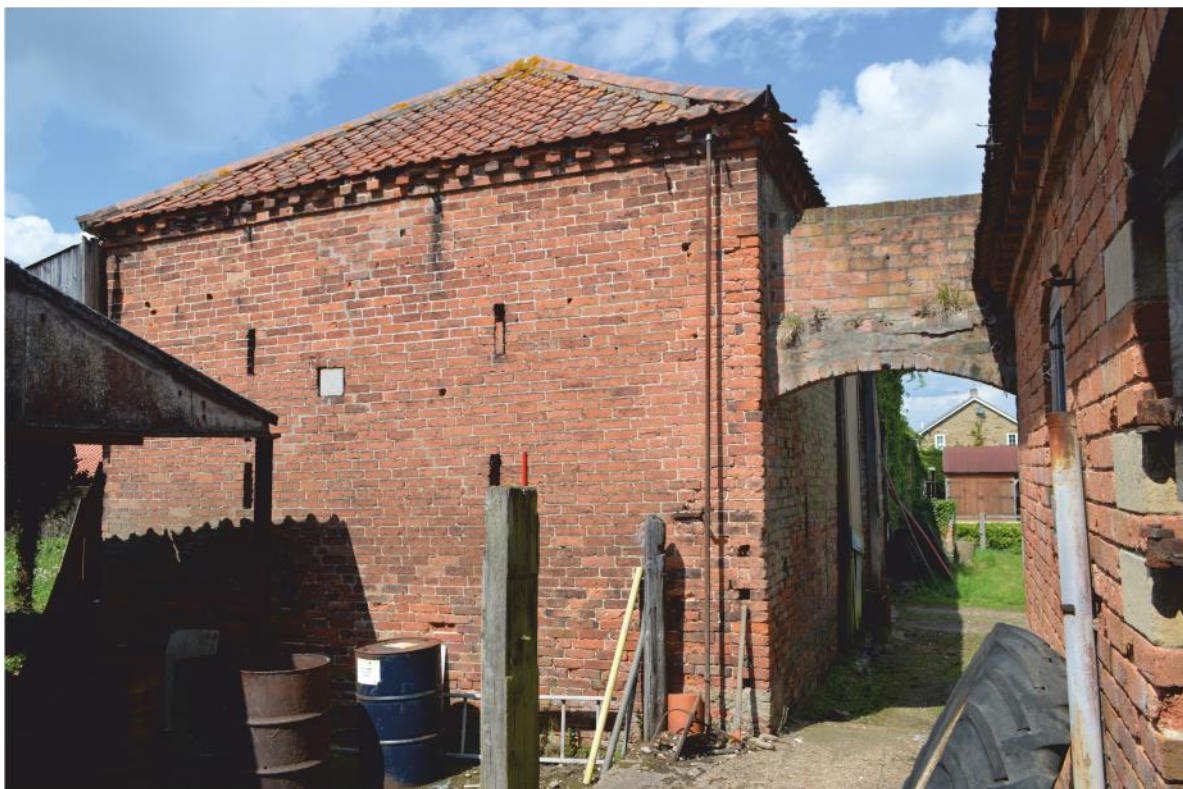
Pl. 46 Building 7, threshing barn, south-east gable
