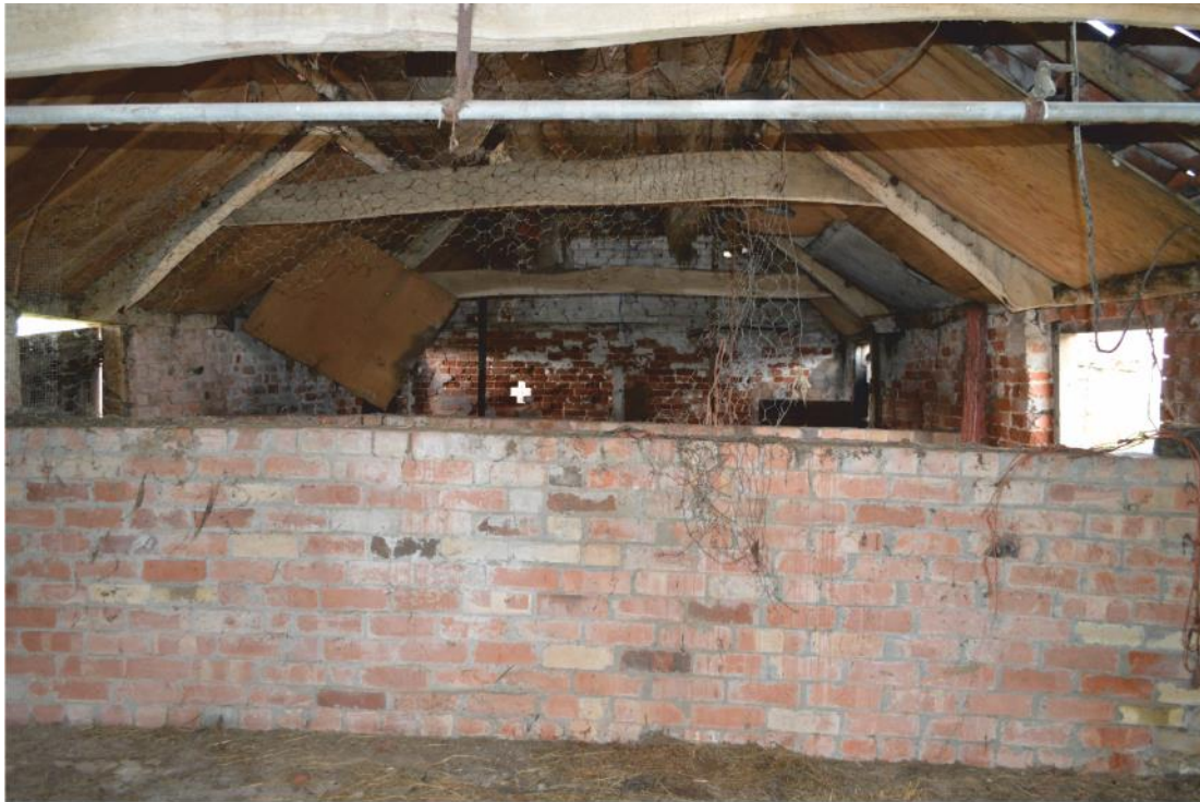
Pl. 25 Building 3 looking south-east
