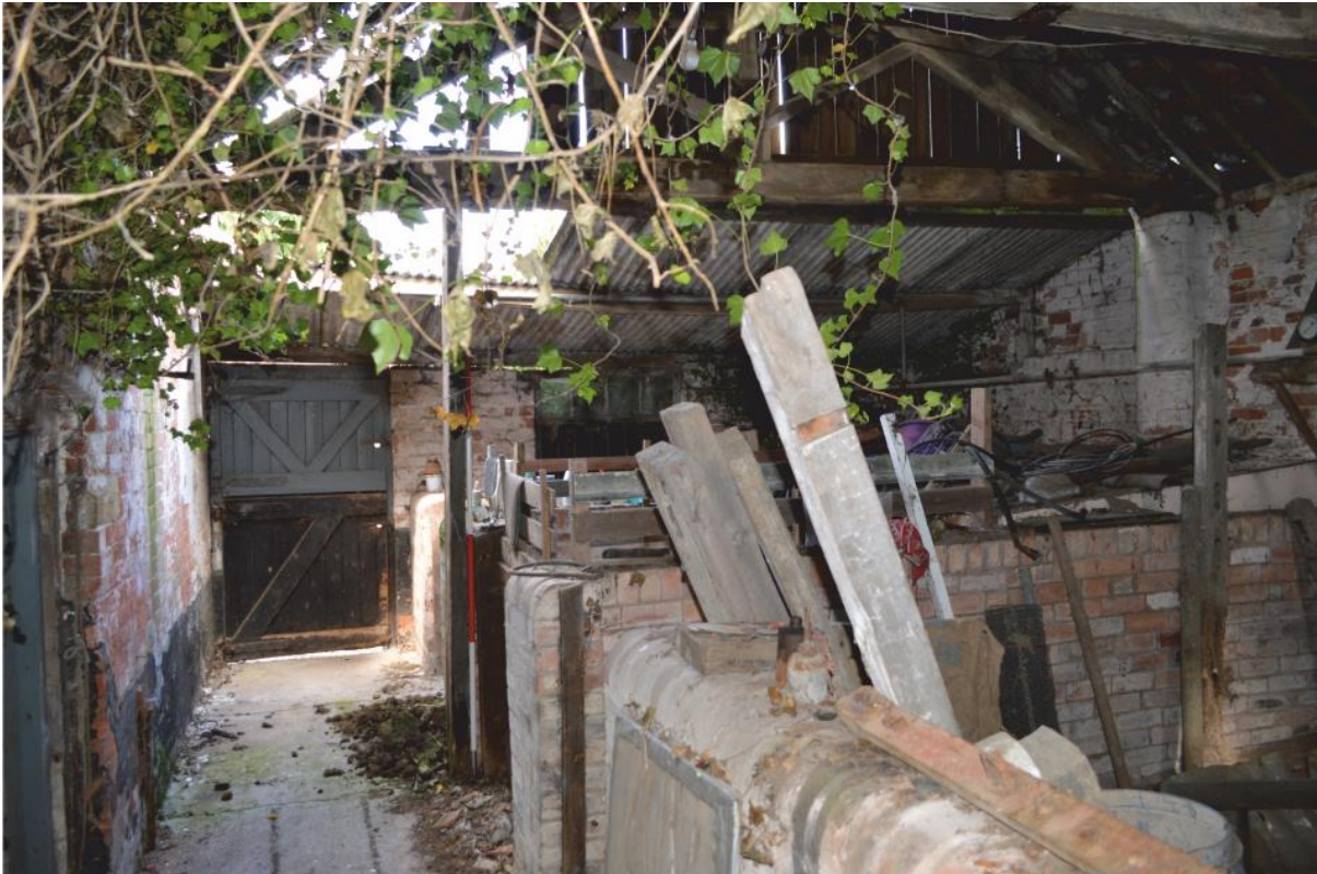
Pl. 53 Building 8 looking north-west
