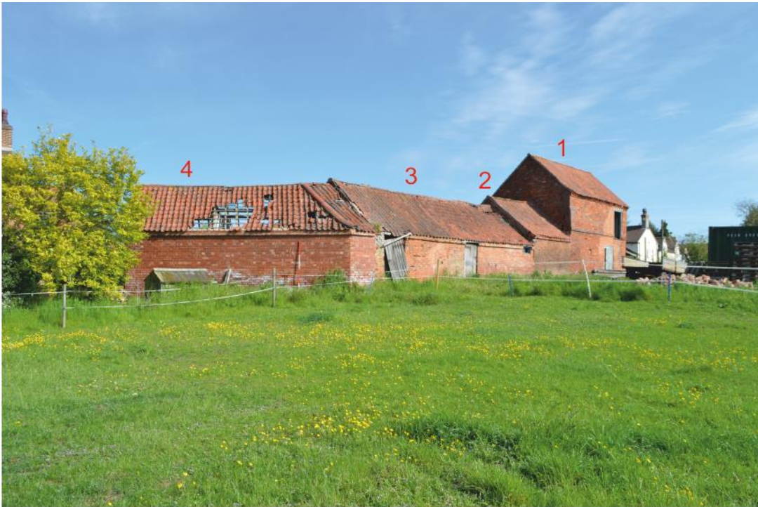
Pl. 3 General view of site looking north, showing buildings 4,3,2,1
