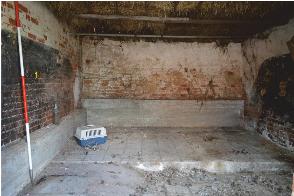
Pl. 20 Building 2 interior, concrete floor and feeding trough to rear
