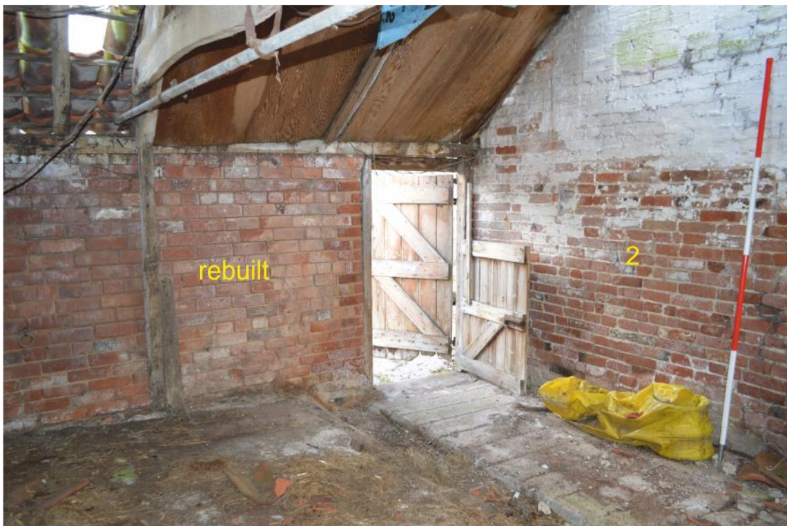
Pl. 24 Building 3 internal view of north door out to the crewyard
