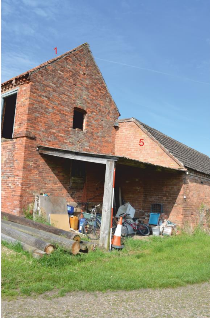
Pl. 9 Building 1 north gable and lean-to
