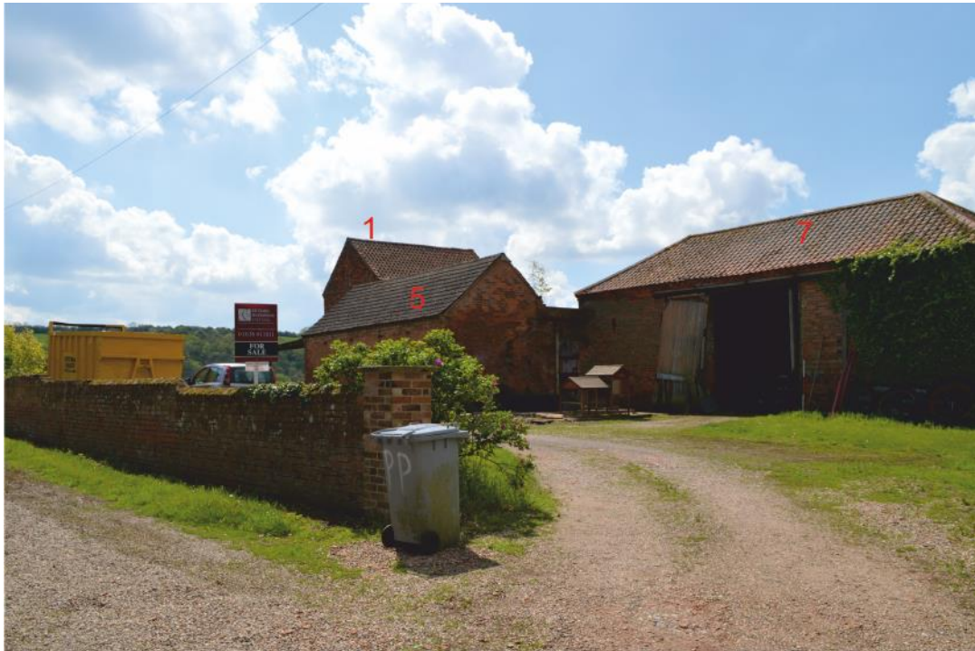
Pl. 1 General view of site looking south, showing entrance and buildings 1,5,7
