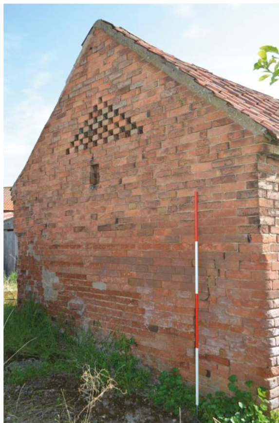
Pl. 30 Building 4 south-west gable, with chamfered angles
