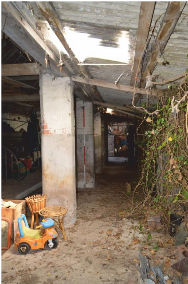
Pl. 62 Building 10, extension to 9, looking north-east
