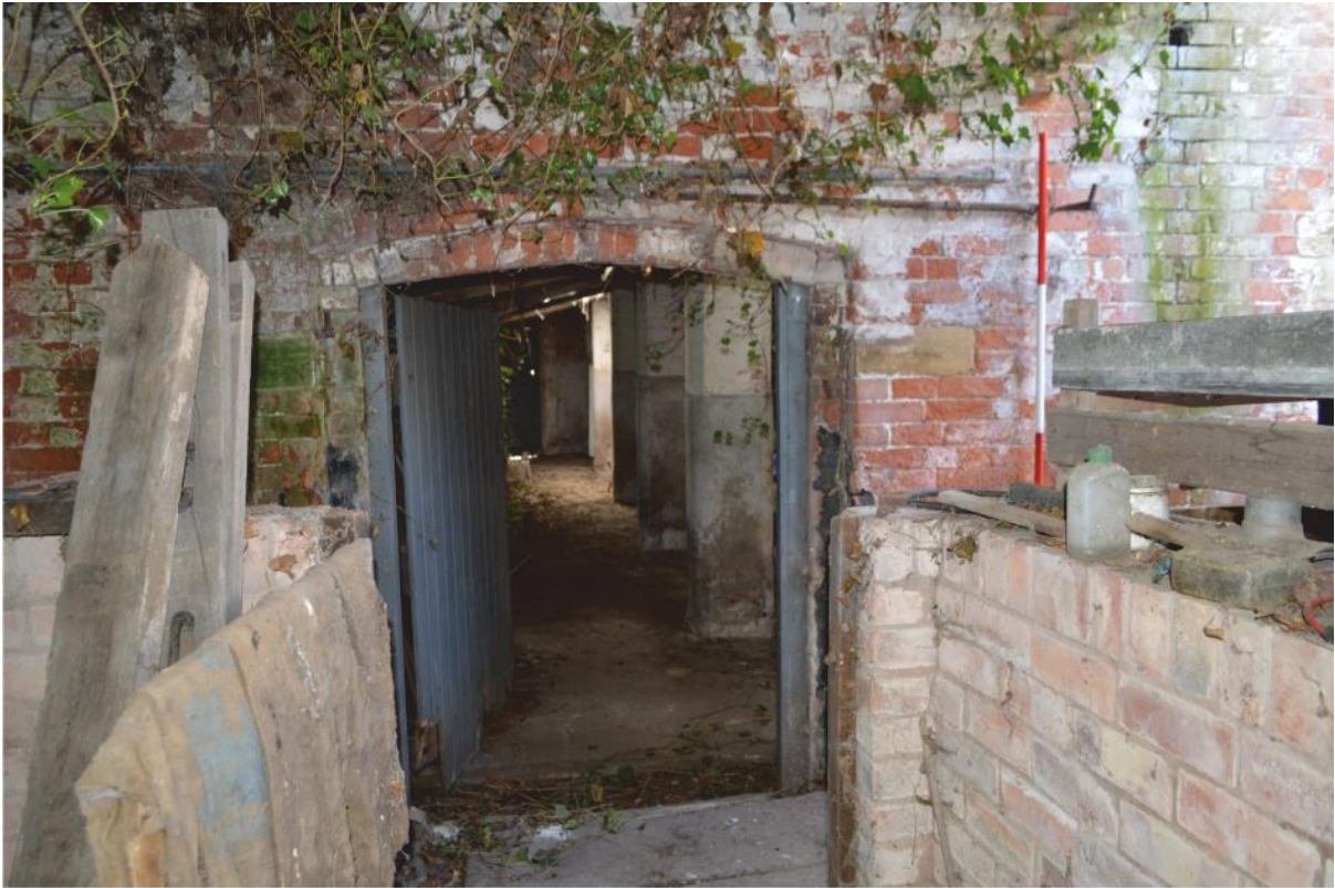
Pl. 57 Building 8, original external access to crewyard (now leads into milking shed 10)
