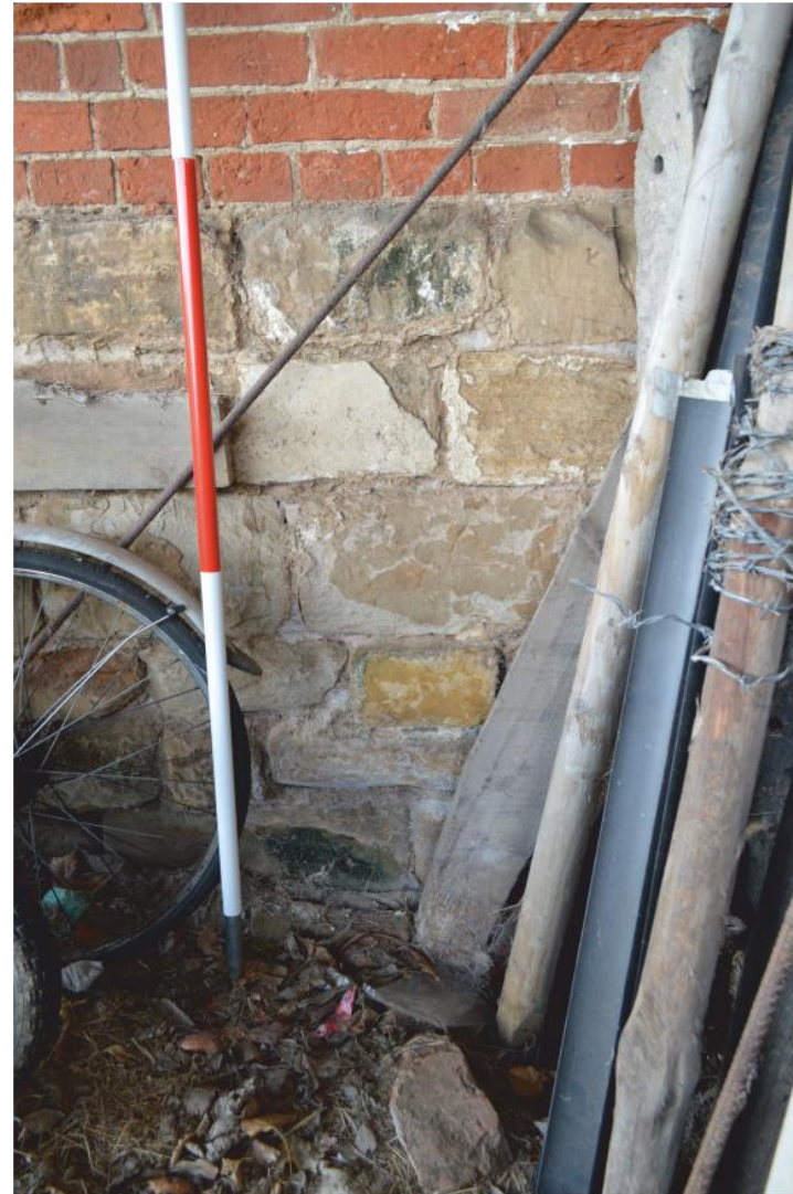
Pl. 10 Stone foundation at base of north gable
