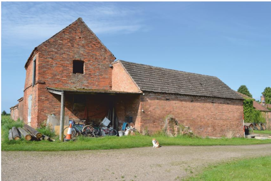
Pl. 34 Building 5 north elevation
