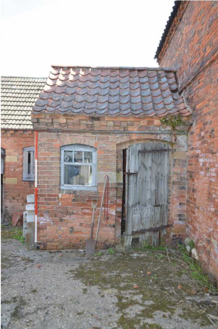
Pl. 41 Building 6, looking north-west
