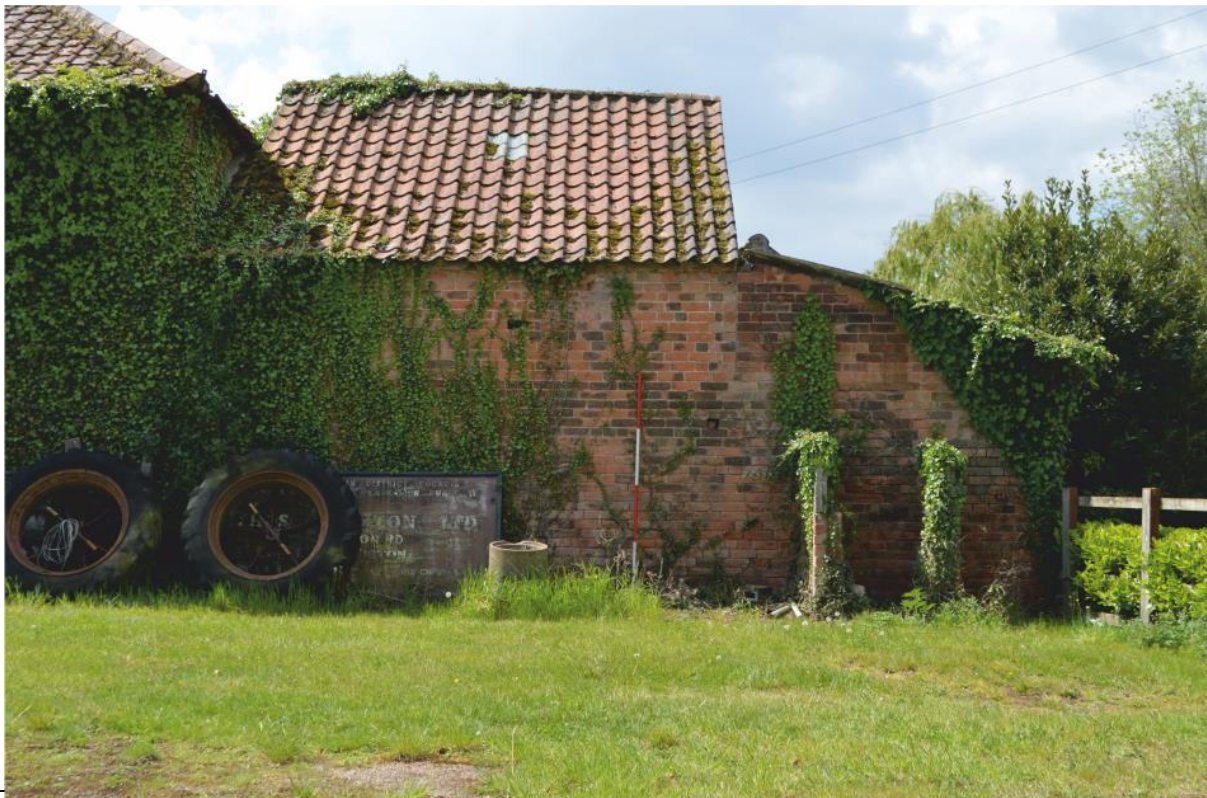
Pl. 52 Building 8 north-east elevation
