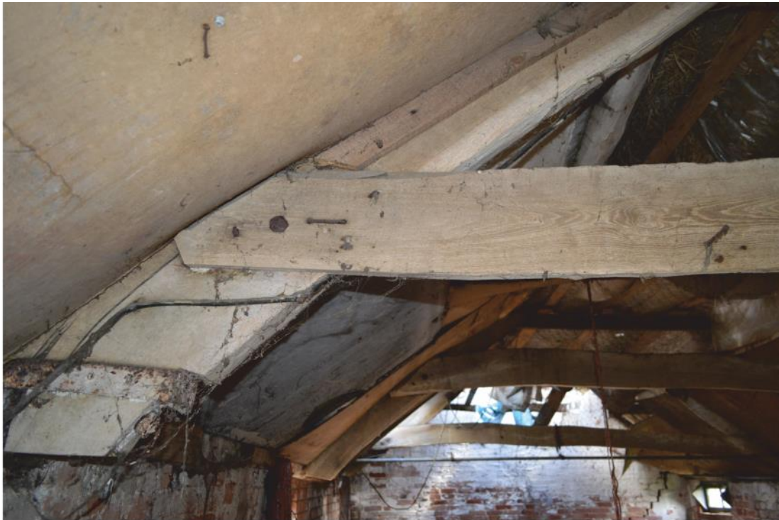
Pl. 27 Building 3 detail of nailed roof truss
