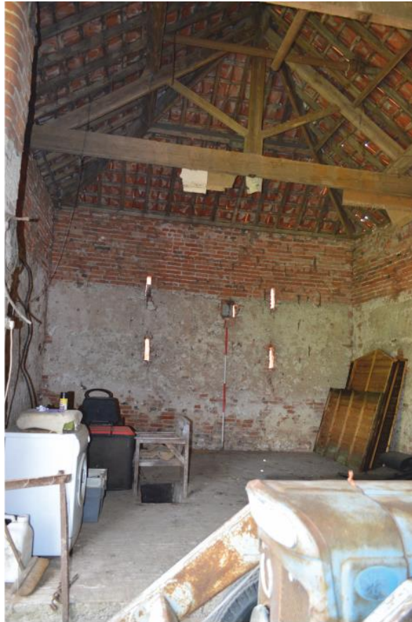
Pl. 49 Threshing barn 7 south-east gable showing hipped roof
