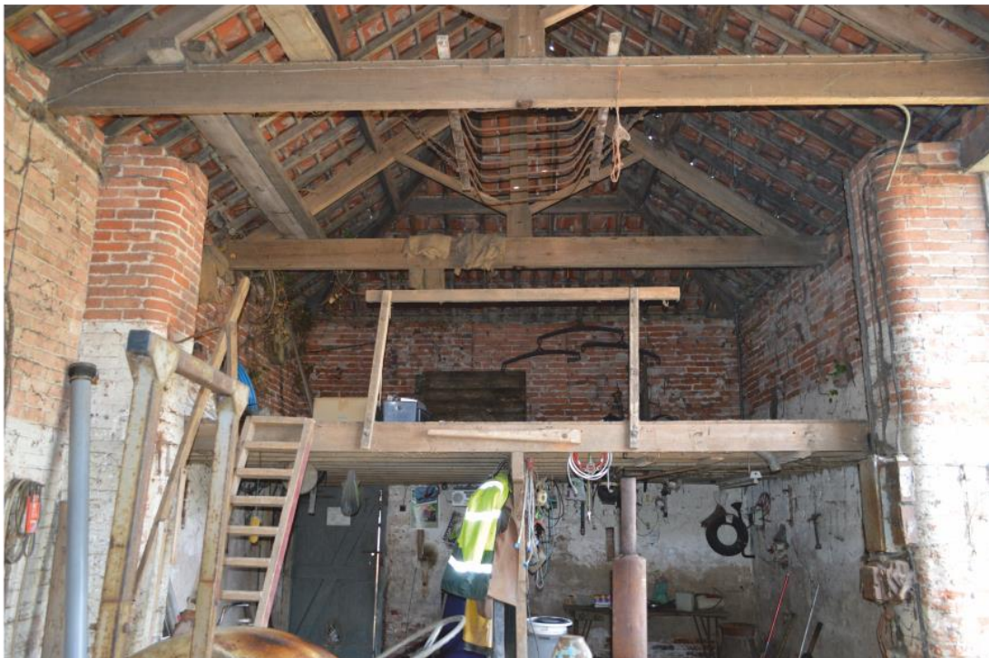
Pl. 50 Threshing barn 7, north-west gable showing hay loft above, access to 8 below.
