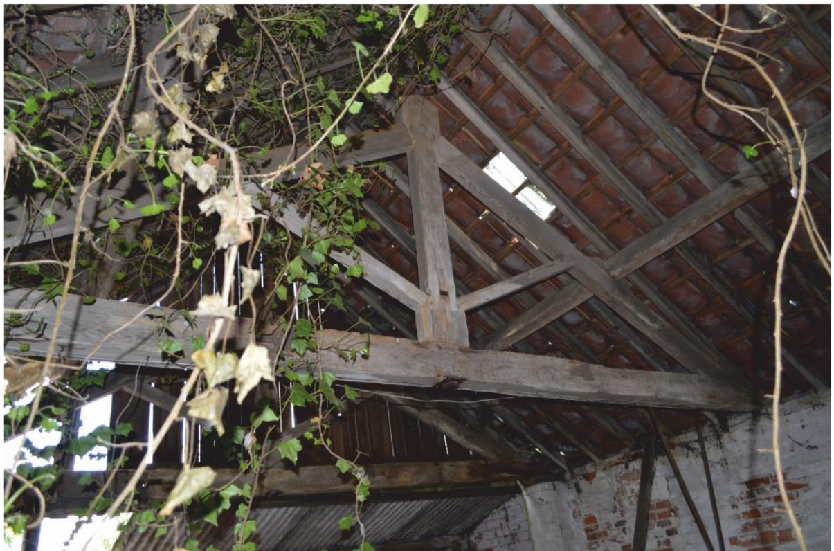
Pl. 54 Building 8, bolted roof truss of machine-sawn timbers
