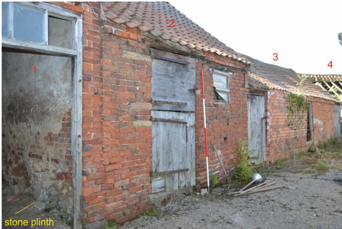
Pl. 19 Building 2 external elevation facing the crewyard
