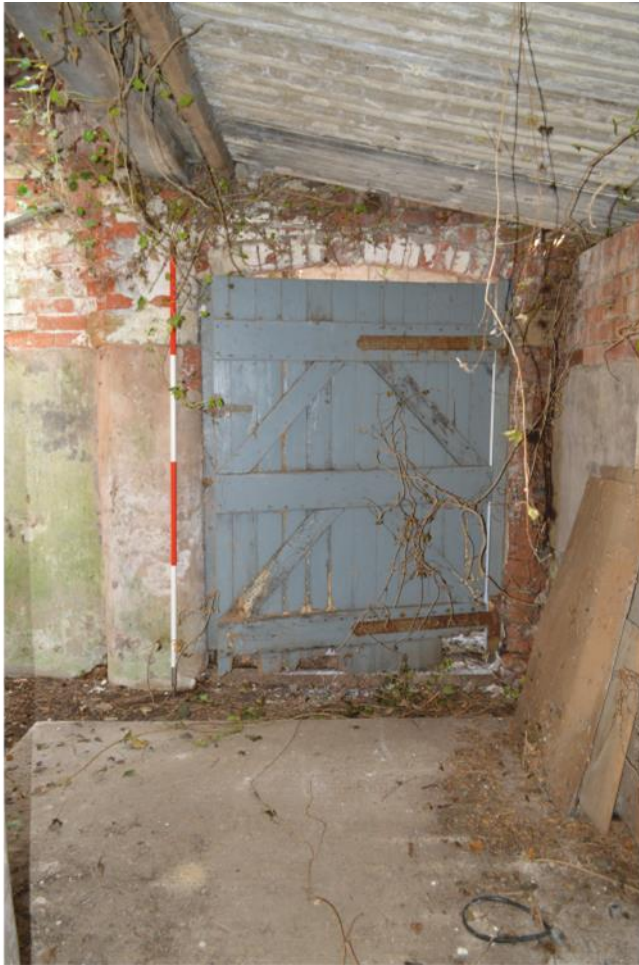
Pl. 63 Door from milking shed into crewyard, looking east.
