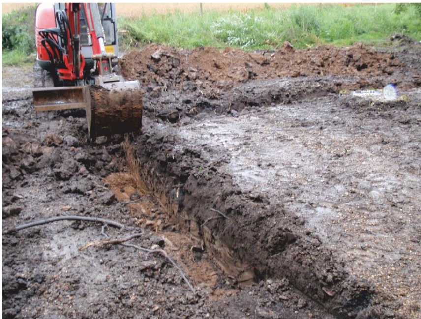
Pl. 2 Excavation of foundation trench in progress, looking east.
