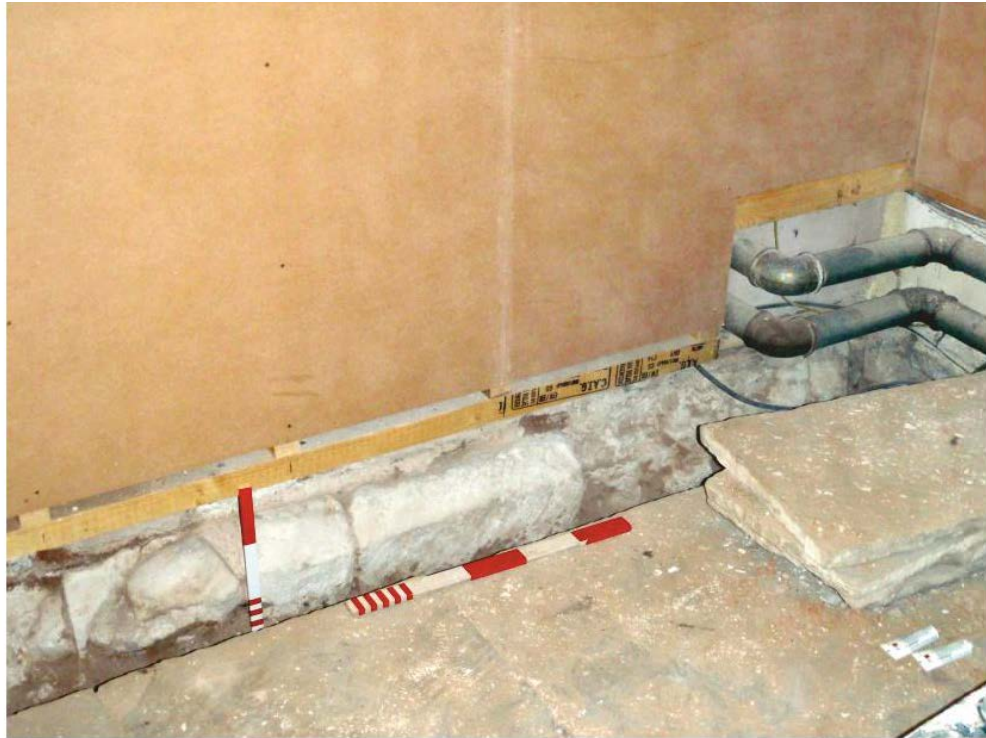
Pl. 3 Plinth at base of tower north wall showing diagonal tool marks on the undamaged stonework. Scales 0.50m and 0.30m.
