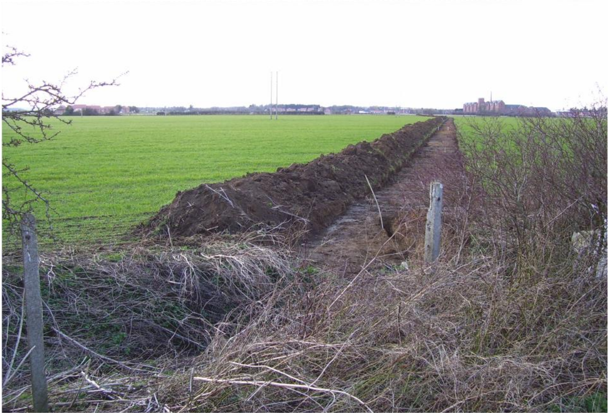
Pl. 5 View from east end of rising main easement, looking west
