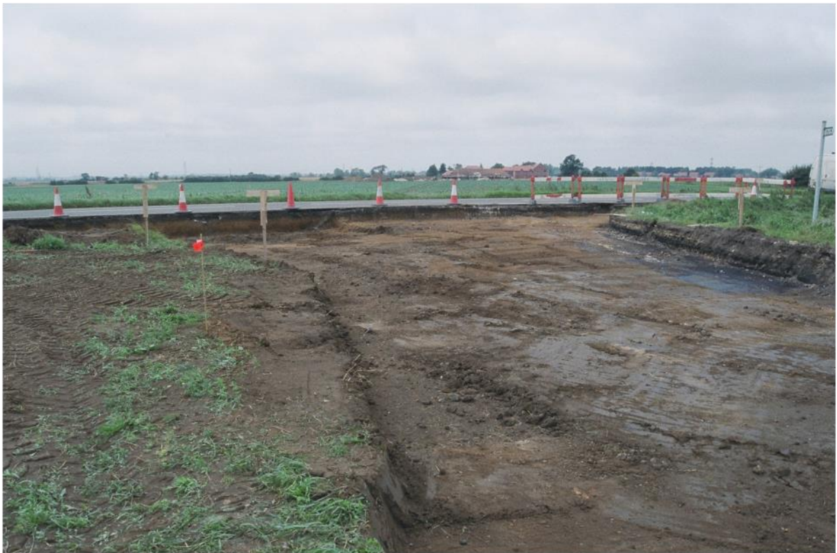
Pl. 2 Entrance to access road off Mareham Lane after stripping, view west.
