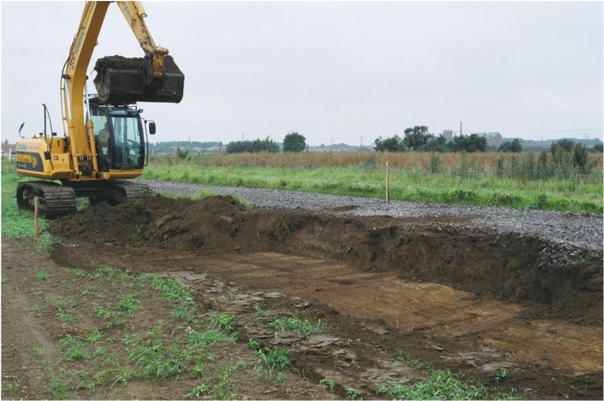
Pl. 3 Stripping in progress, view north-west.
