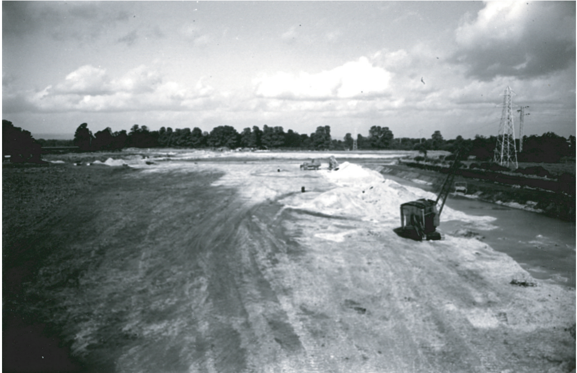
Figure 14: general view of Netherhills Quarry in 1948
