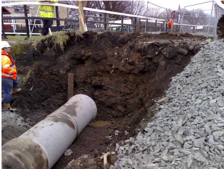
Figure 18: The dog legged pipe from the W Inlet Chamber looking NE
