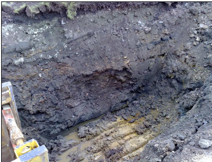
Figure 19: A typical section of the W portion of the pipe track
