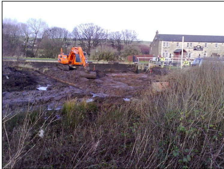
Figure 8: Looking NNE at the re-routed water course (running SE-NW)
