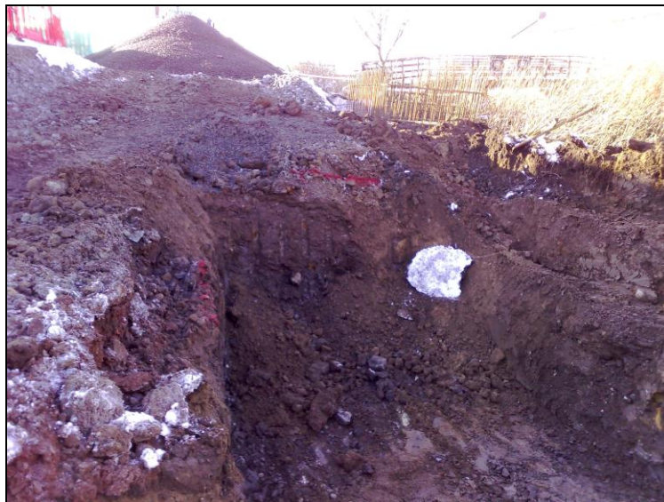
Figure 14: Looking E at Trench 3 for the E Baffle Chamber
