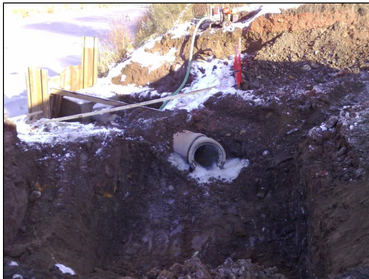
Figure 7: Looking NE at the completed E Outlet Chamber with fitted Pipe
