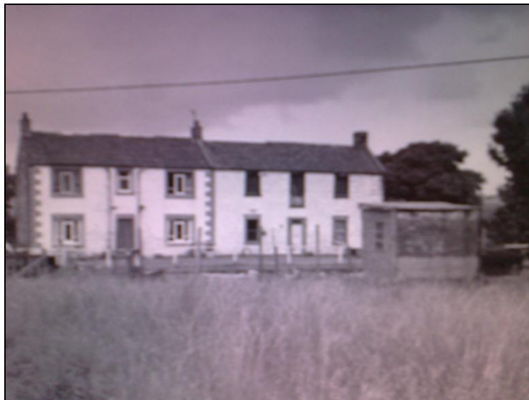
Figure 21: The brick outhouse on the S side of Lock 17 looking NNE c.1970s
