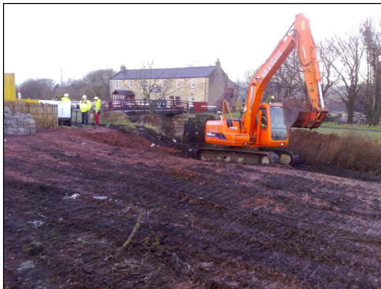
Figure 3: Remains of the Blaze Dam looking NW
