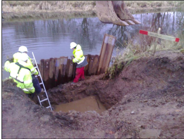
Figure 6: Trench 1 and the Cofferd Dam looking NNE
