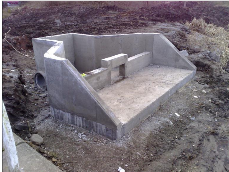
Figure 13: The W Inlet Chamber looking SW
