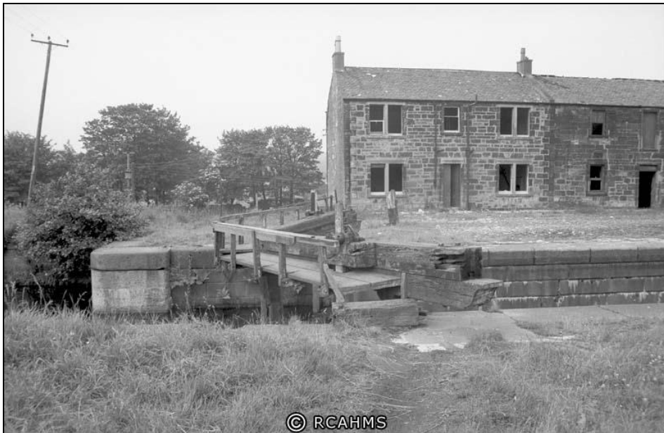
Figure 6: View of 1970 from SSE showing top of W lock gates with part of lock keeper's house and stables in background (RCAHMS SC733396)
