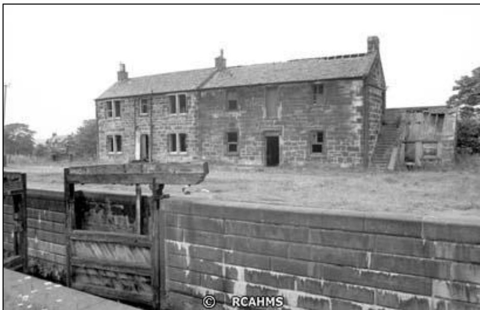
Figure 7: View of 1970 from SE showing SSE and ENE fronts of lock keeper's house and stables with remains of E lock gates in foreground (RCAHMS SC733397)
