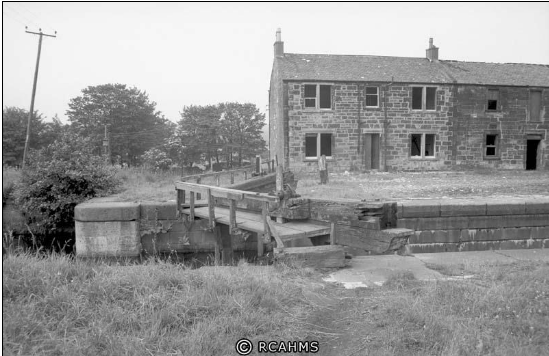
Figure 6: View of 1970 from SSE showing top of W lock gates with part of lock keeper's house and stables in background (RCAHMS SC733396)
