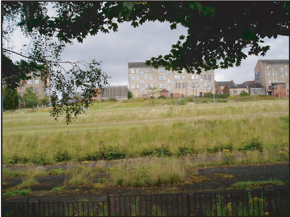
Plate 9: Tenement buildings from west
