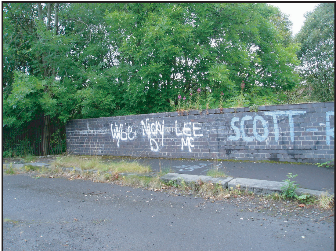
Plate 8: Remains of Bridge (Site 61) from north east
