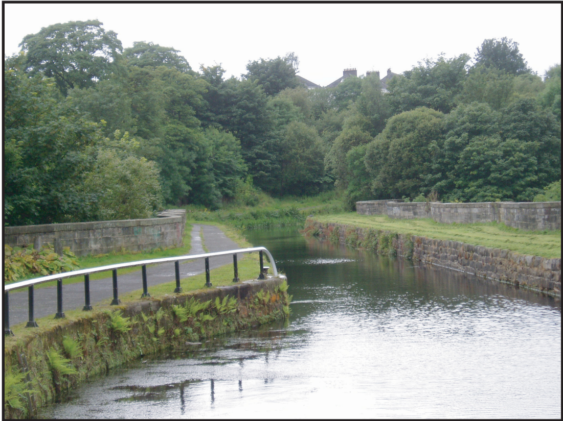
Plate 3: Kelvin Aqueduct from west
