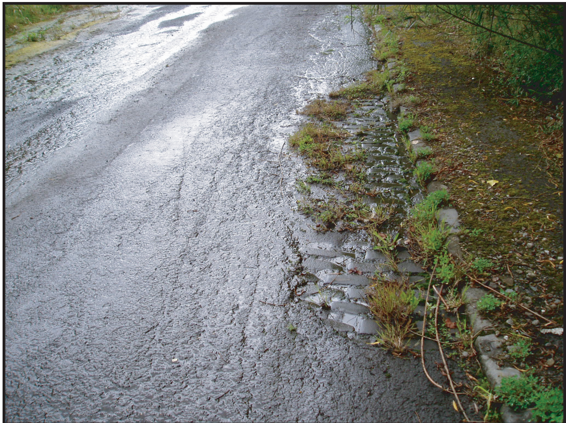
Plate 4: Cobbled surface visible beneath tarmac from west
