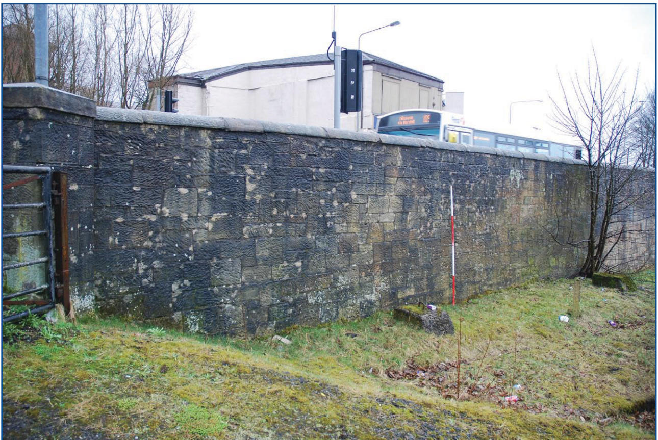
Plate 26: General view of the eastern wall to Maryhill Road from NW
