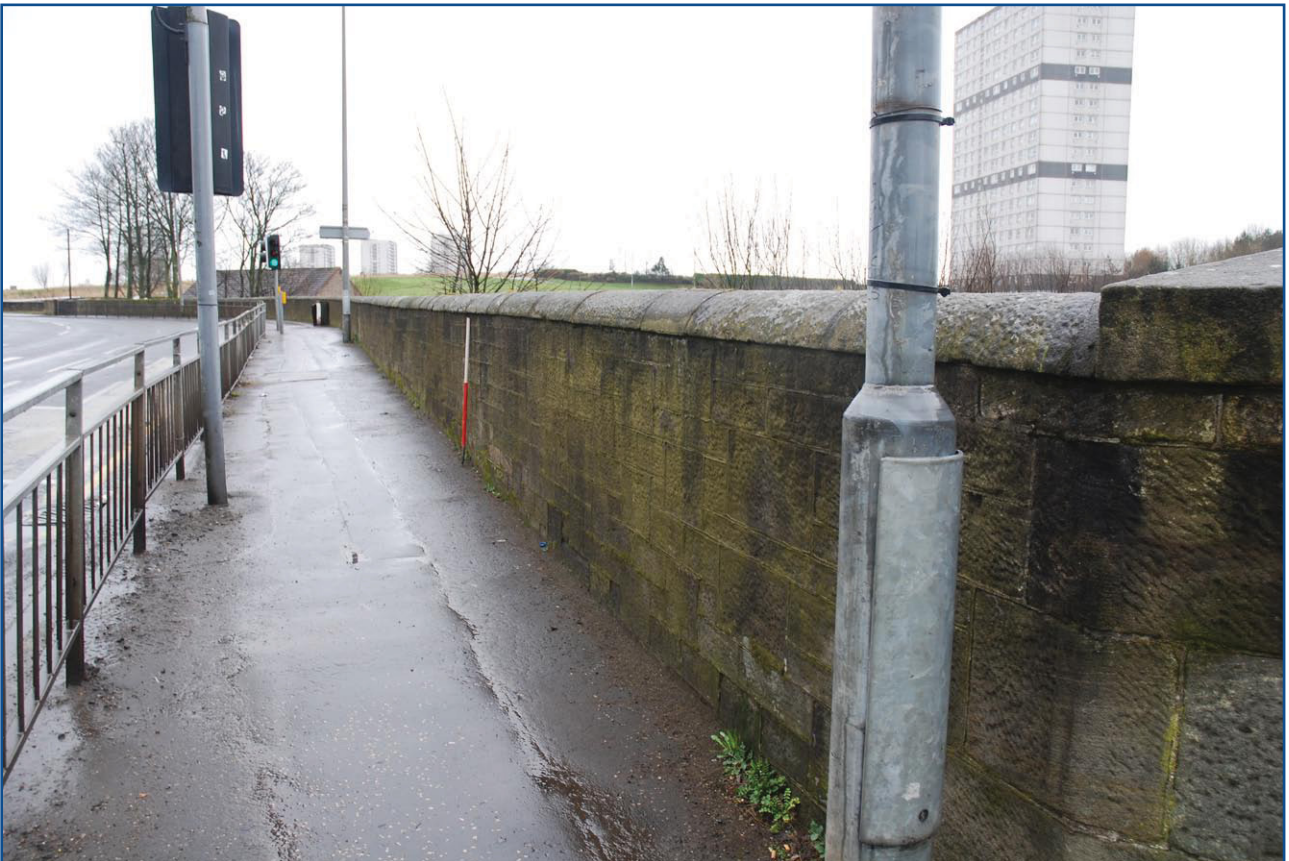
Plate 28: General view of the eastern wall to Maryhill Road from NNE
