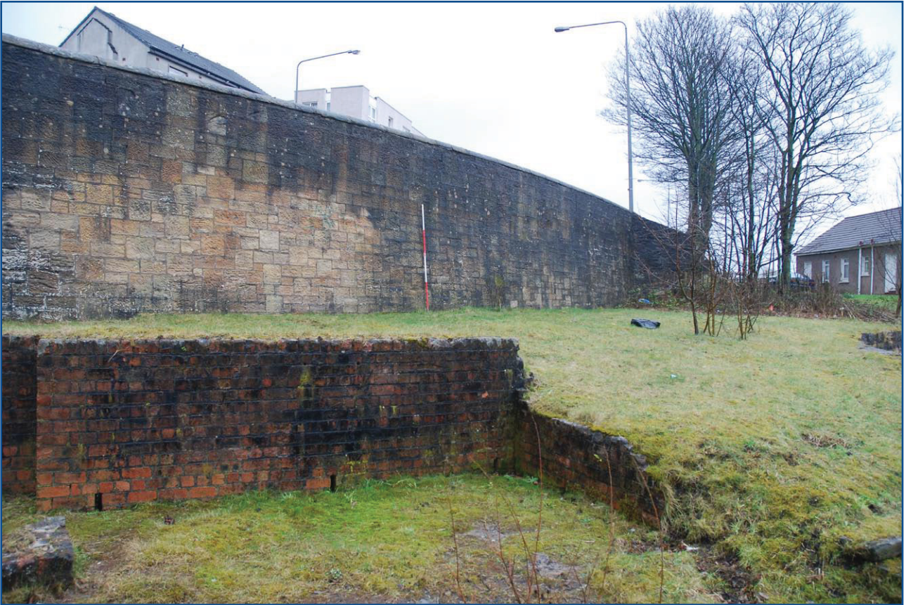
Plate 27: General view of the eastern wall to Maryhill Road from NW
