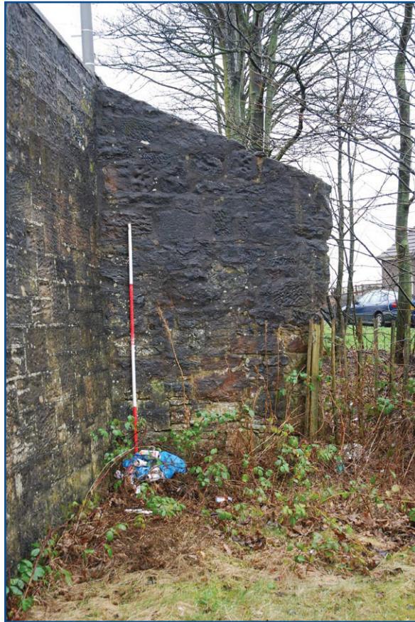
Plate 29: Detail of the stretch of wall on southern side of eastern wall to Maryhill Road
