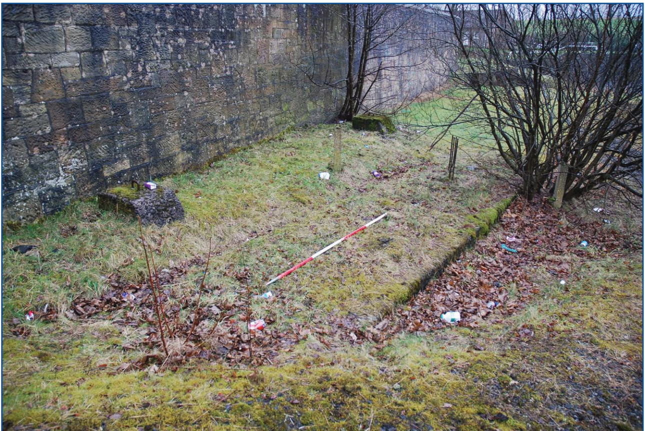
Plate 30: General view of the northern side of the slipway, showing concrete footings and associated fittings from NW
