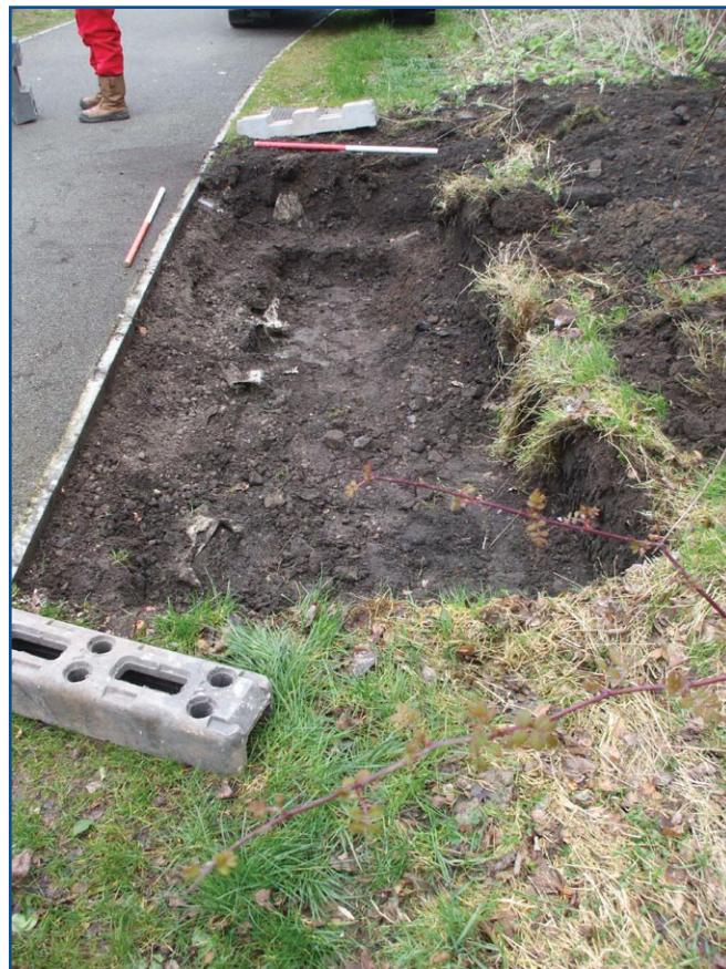
Plate 10: Trench 5 from west
