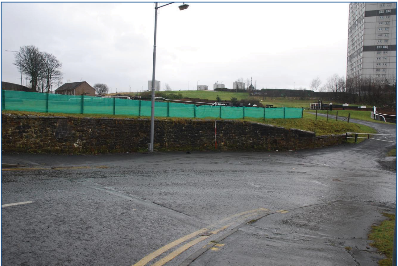
Plate 24: General view of the north wall to Skaethorn Road from NE
