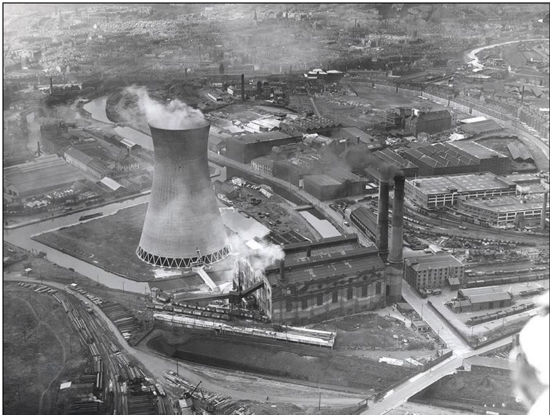
Figure 9: The Pinkston Basin and Cooling Tower, c.1950's
