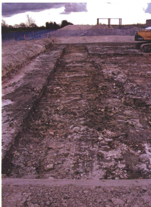
Plate 1 Looking east across trial trench
