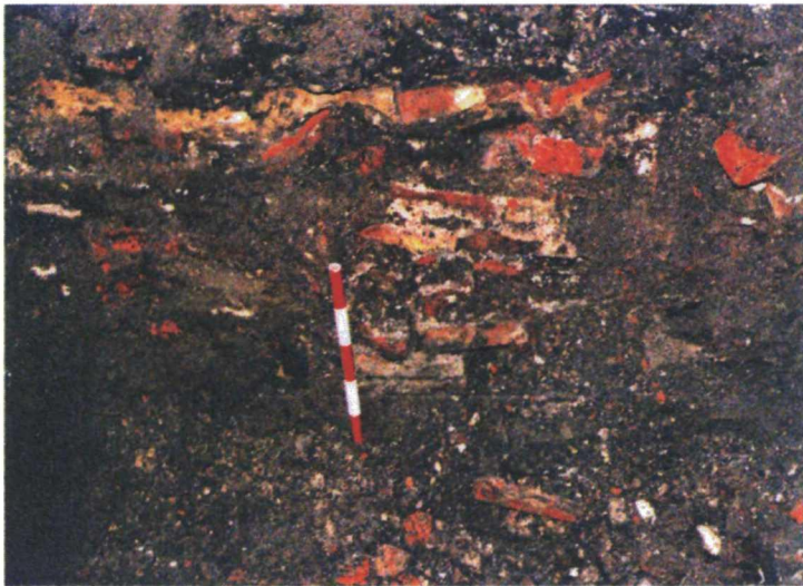
Plate 1 Section through Wall 99012, looking south-west
