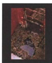
PID: 11861 (1057-42 - print 2004-62-04) Eastern access road. Base of sewer trench. (62978 bytes)
