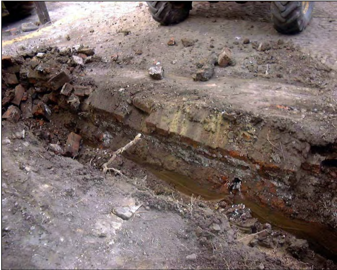
Plate 1. Trench 1, east/west oriented brick wall foundations (102) from the southern elevation of Unit B.
