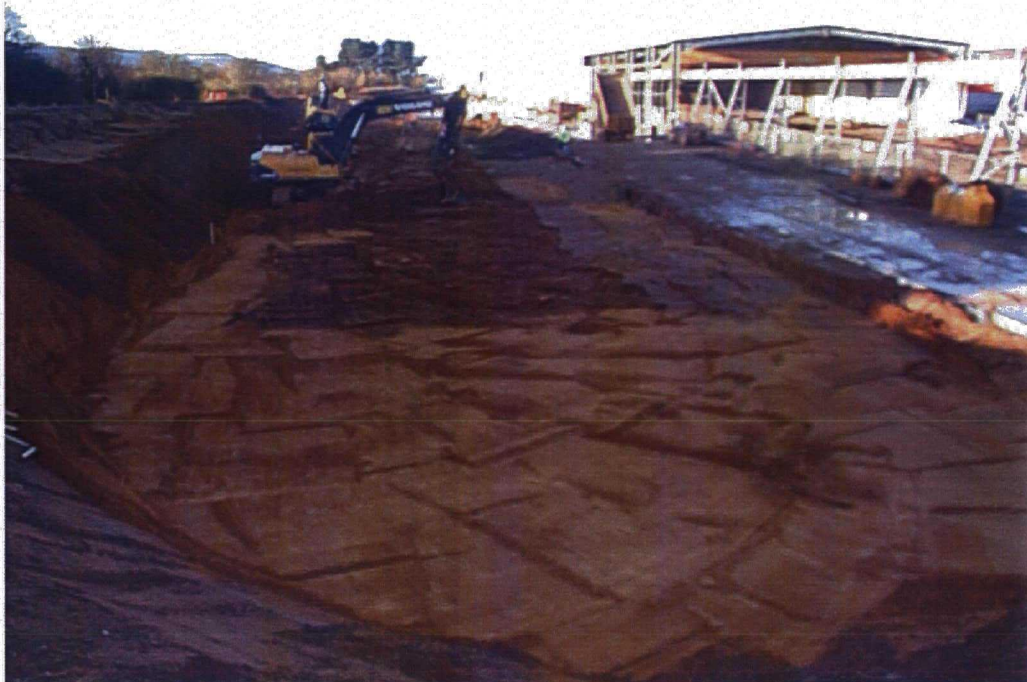
Plate 6. Eastern End of Excavation showing Deposit 1009. Facing West
