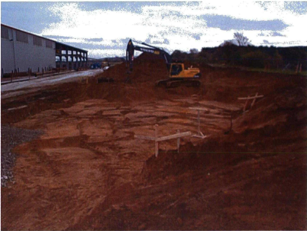
Plate 2. General View of Excavation. Facing East
