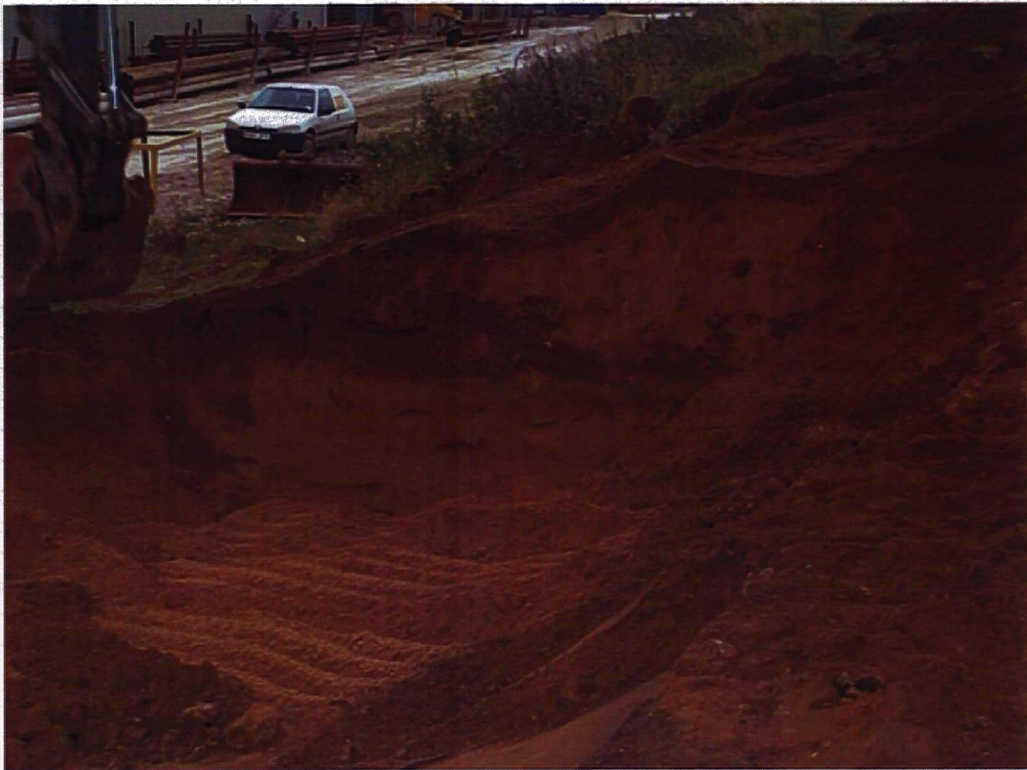
Plate 5. Working Shot showing Deposits 1003 and 1001. Facing East
