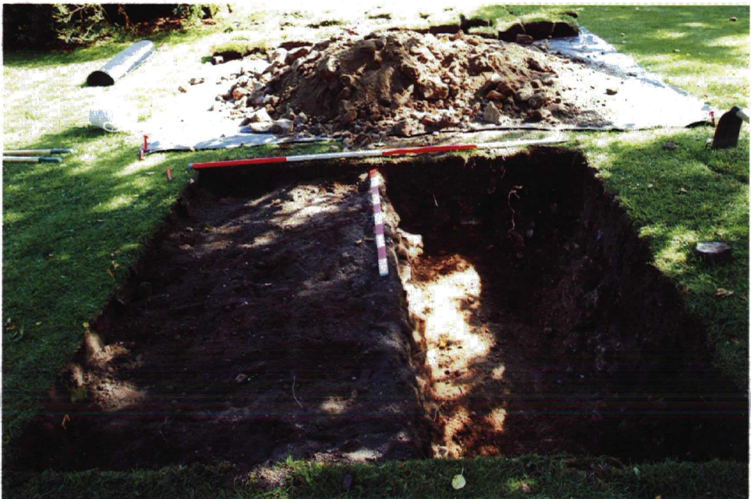
Plate 15: Post-excavation view of Trench 8 from north (Scales = 1m & 2m)
