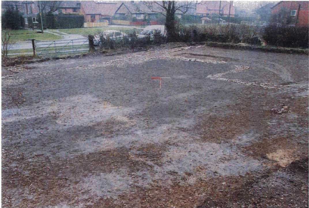
Plate 1. View of Site after Removal of Topsoil and Subsoil. Facing South West
