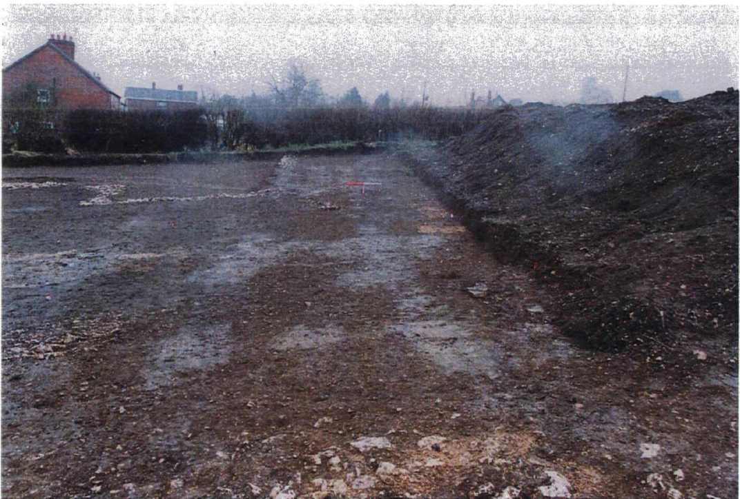
Plate 2. View of Site after Removal of Topsoil and Subsoil. Facing West
