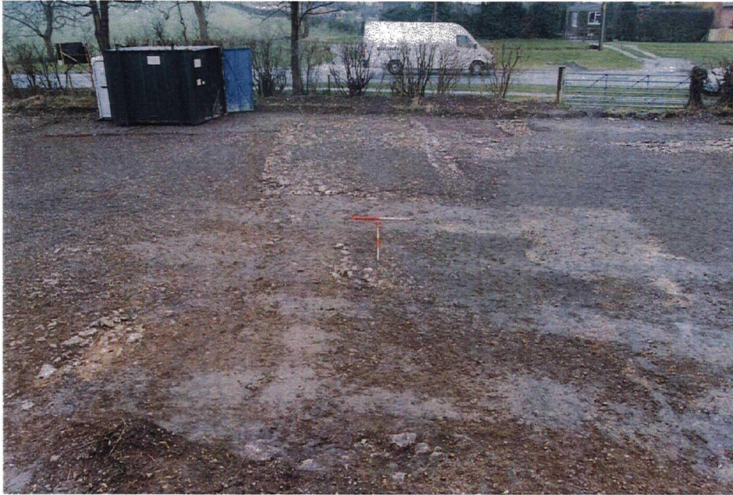
Plate 3. View of Site after Removal of Topsoil and Subsoil. Facing South
