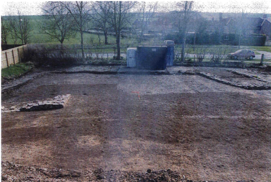
Plate 10. View of Site after removal of Rubble Spreads. Facing South
