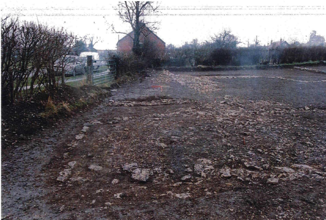
Plate 4. View of Site after Removal of Topsoil and Subsoil. Facing West
