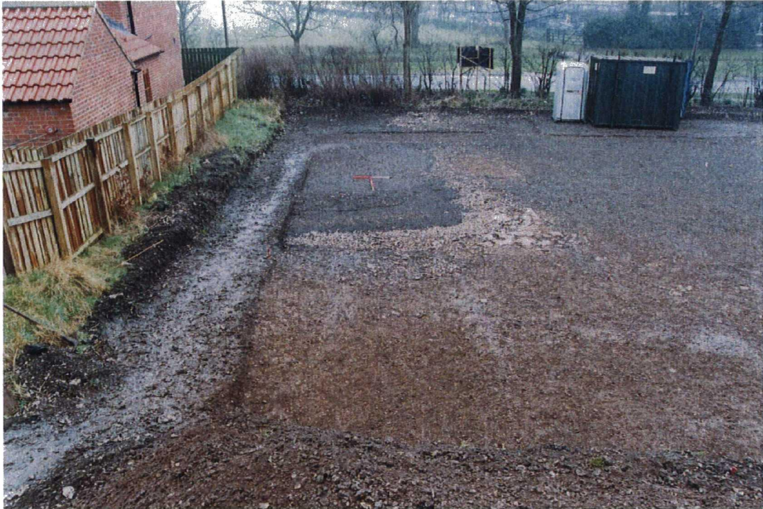
Plate 5. View of Site after Removal of Topsoil and Subsoil. Facing South
