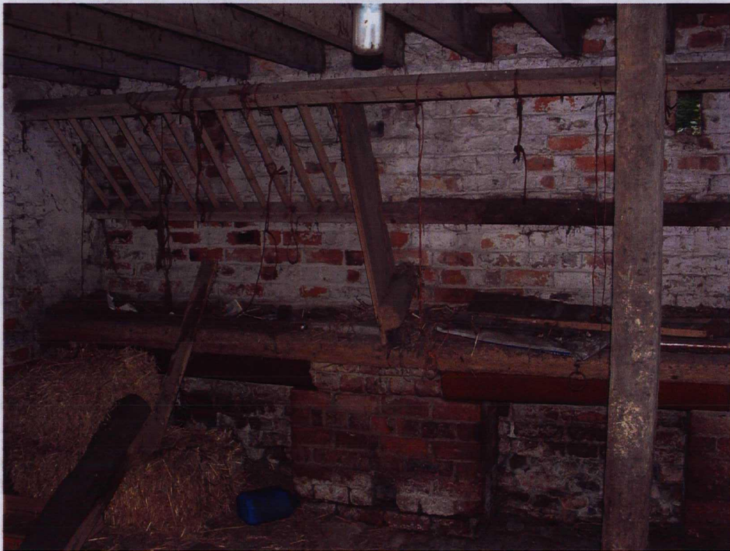
Plate 10 - Central ground-floor room in nineteenth-century agricultural building. Manger, drinking troughs and tethering rings demonstrates recent use as a stable.
