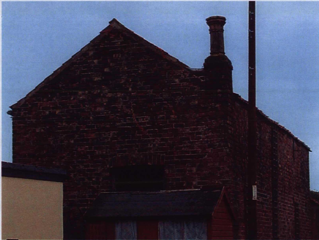
Plate 9 - North face of building shown in Plate 8; note handmade bricks and chimney stack with decorative pot.
