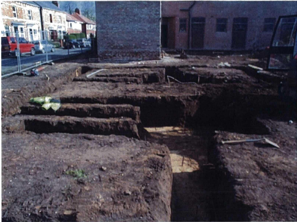
Plate 3. General Working Shot. Facing South
