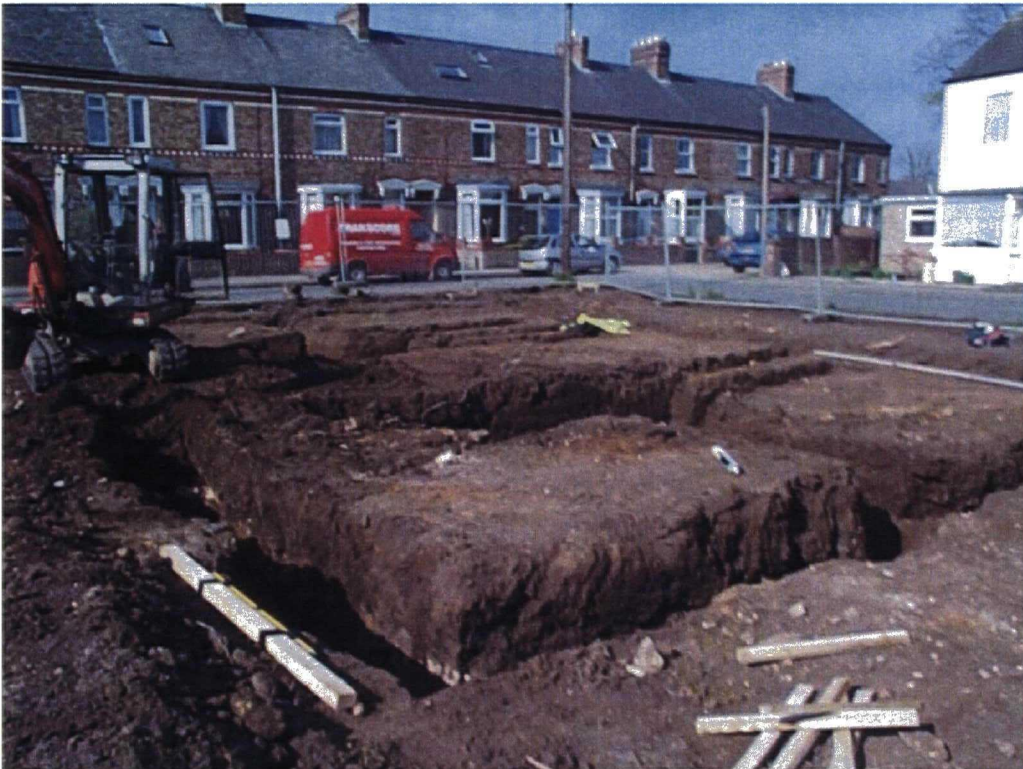
Plate 2. General Working Shot. Facing North East
