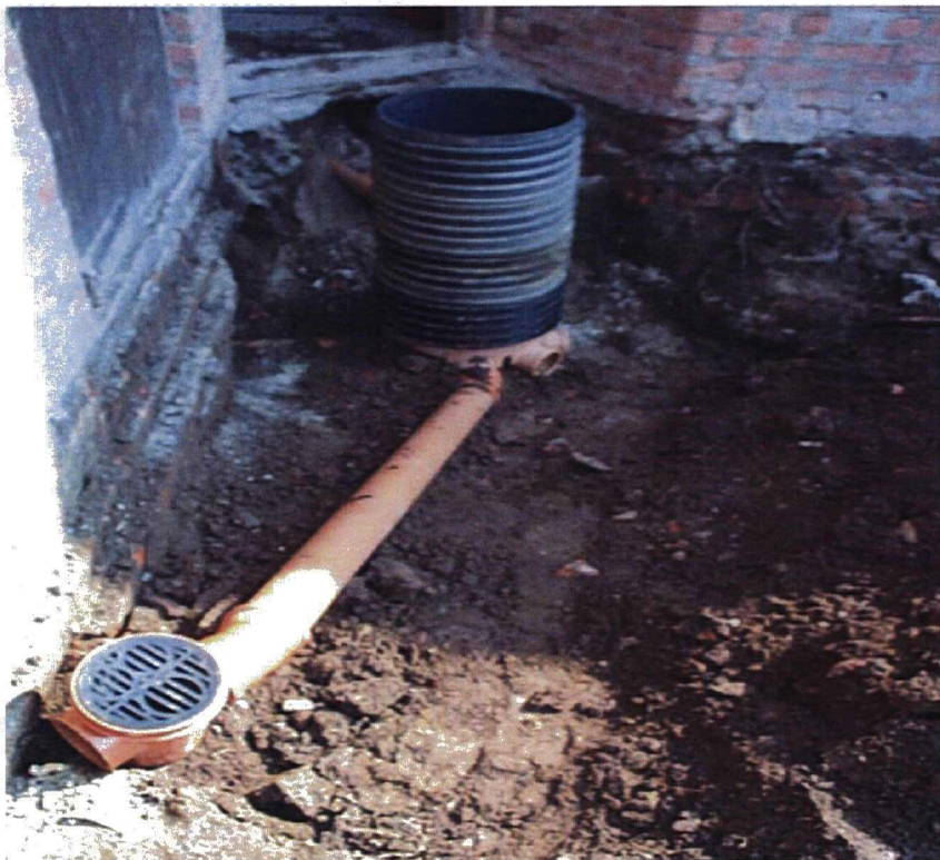
Plate 8. Post-Excavation Photo of Man-Hole Services. Facing South
