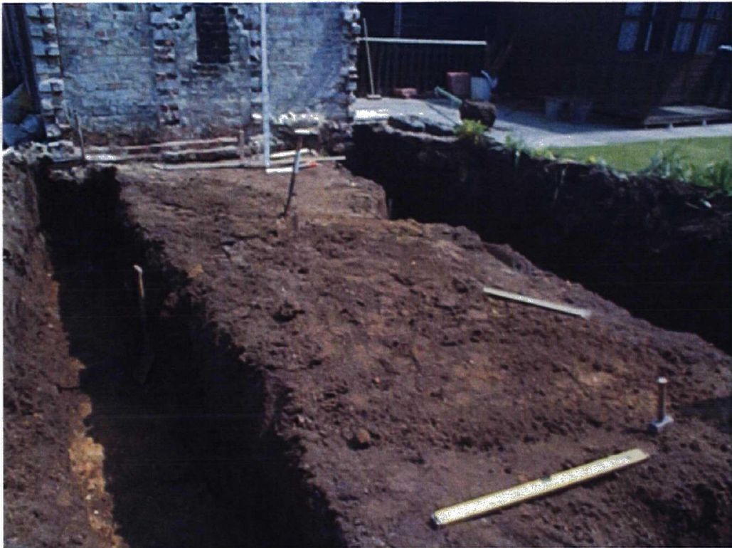
Plate 7. Post-Excavation Photo of Plot 4 Foundations. Facing East
