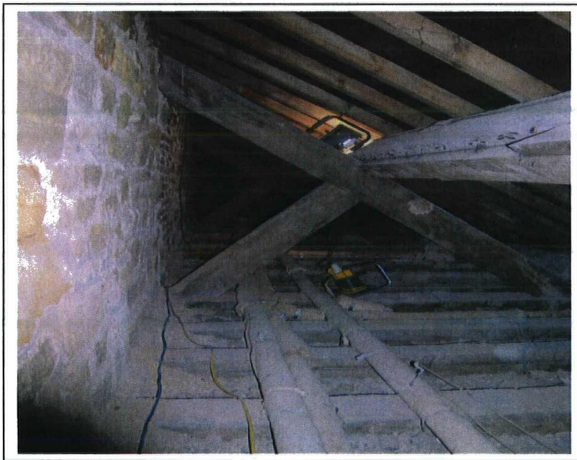
Figure 3a (top): View of a truss from the roof of the main range
