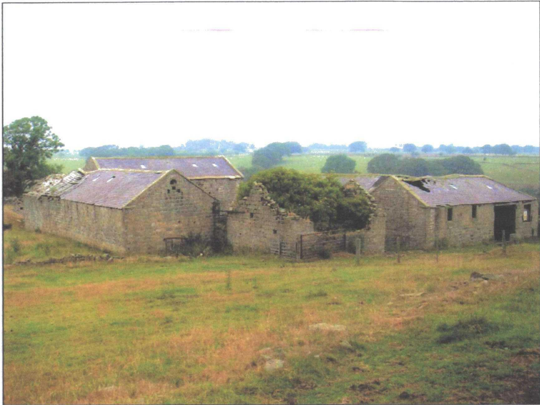
Plate 7. The main range of buildings at Haverah Park Top, looking north-east
