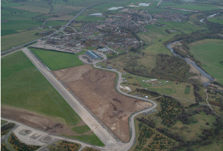
Figure 37 Aerial view of the site © English Heritage
