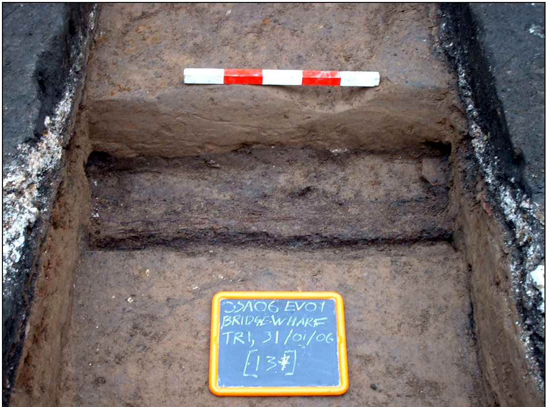
Plate 2. Possible structural slot [137] in trench 1 and in-situ horizontal timber. (Scale of 0.5m).
