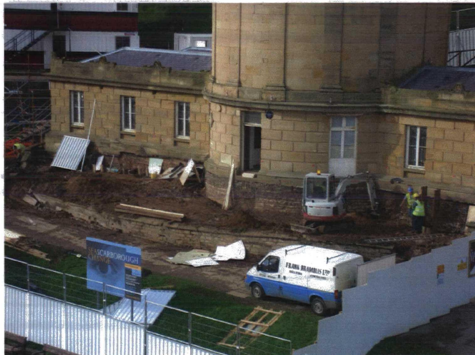
GROUND WORKS IN PROGRESS
