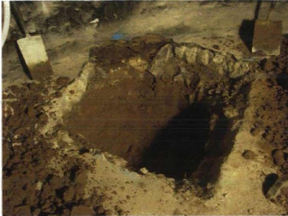
Photograph 1 - Northern trial pit in the cellar Showing modern concrete floor directly overlying undisturbed sandy glacial clay
