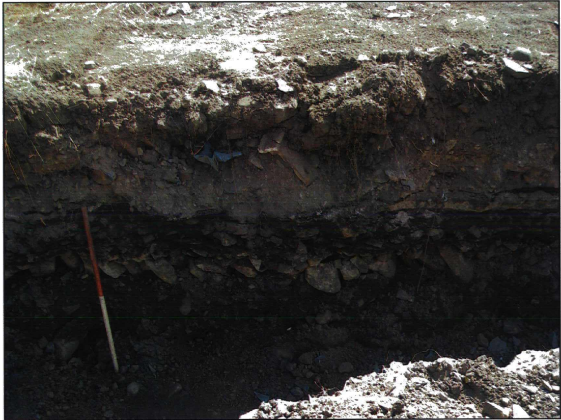
Plate 2: South-eastern corner of Plot 9 showing disturbance by tarmac and hardcore layers; possibly represents a modern road foundation.
