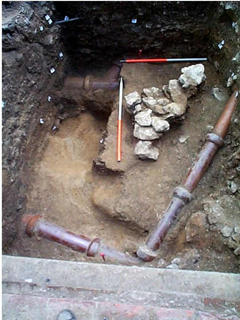
Plate 6. Trench 3. Structure 3013/3025 and Pits 3031 and 3025. Facing South
