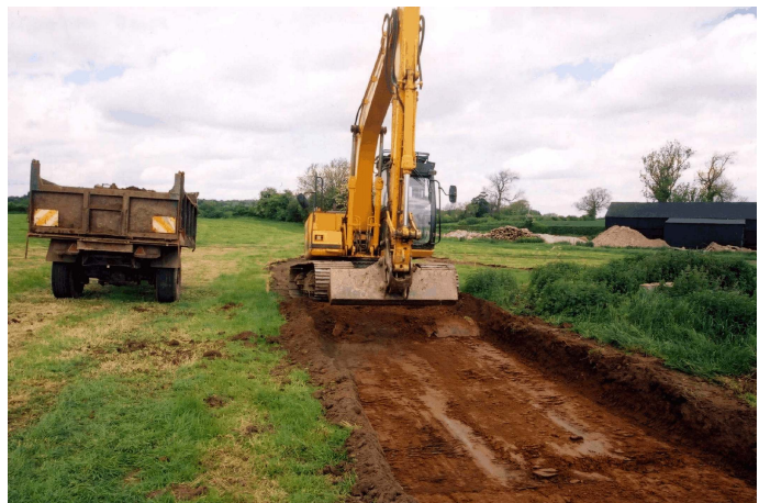
Plate 1 Topsoil removal along access road
