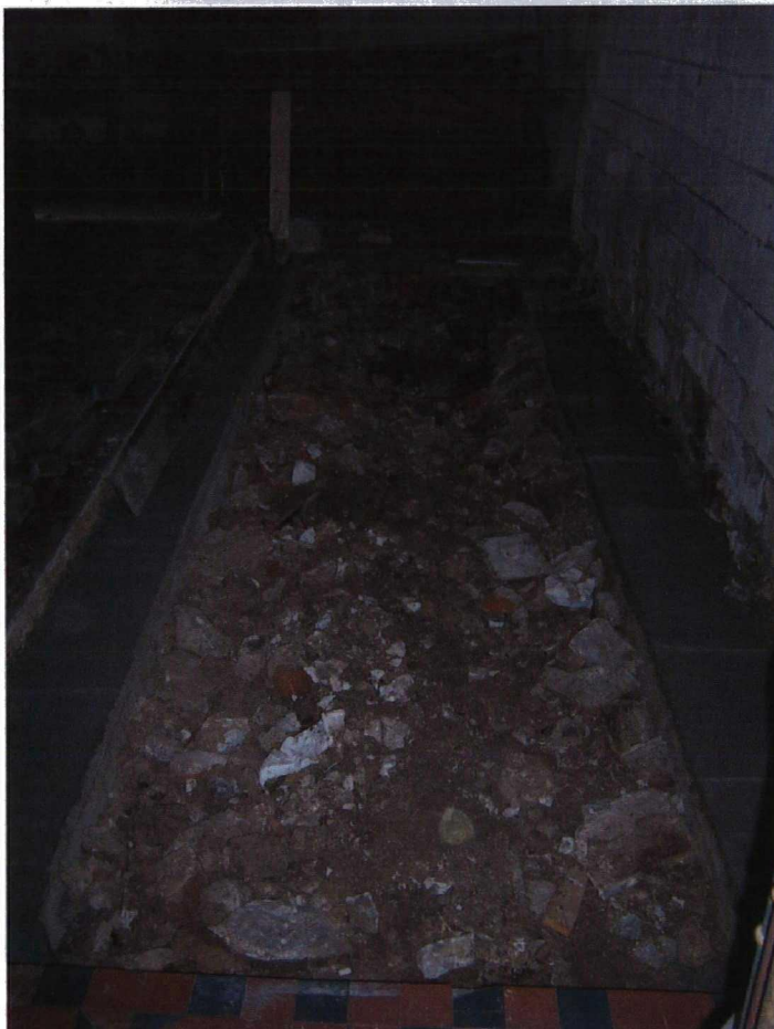
Plate 2 The northern pew area, partially completed, looking west.
