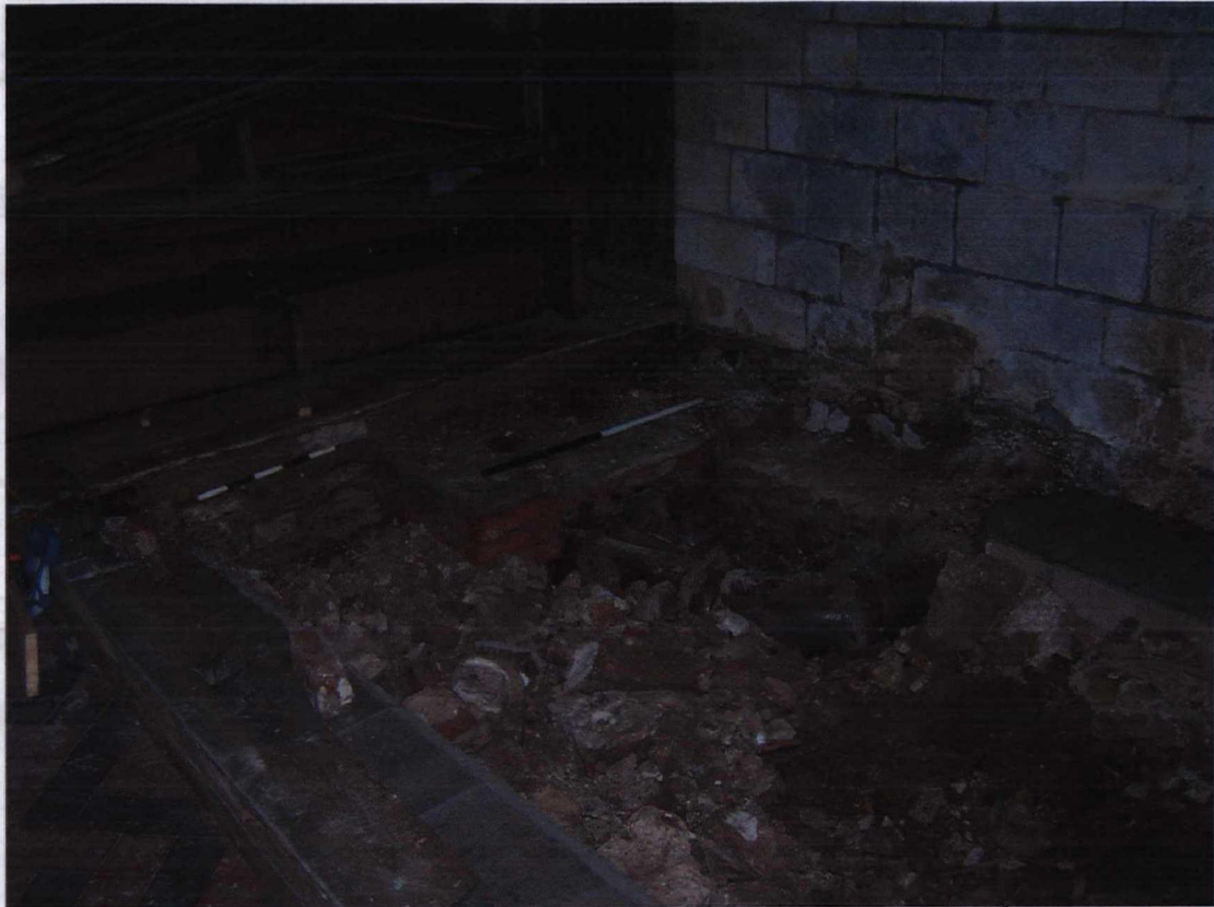
Plate 3 The western end of the northern pews: limestone and chalk foundations, 19 th century services, church foundations and underpinning, modern concrete beams and rubble, looking north-west.
