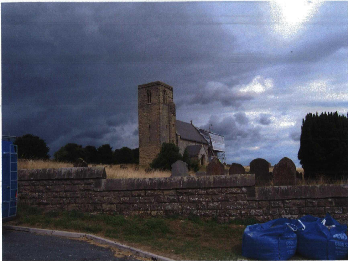
Plate 1 St. Andrew's, Weaverthorpe, viewed from the south-east.
