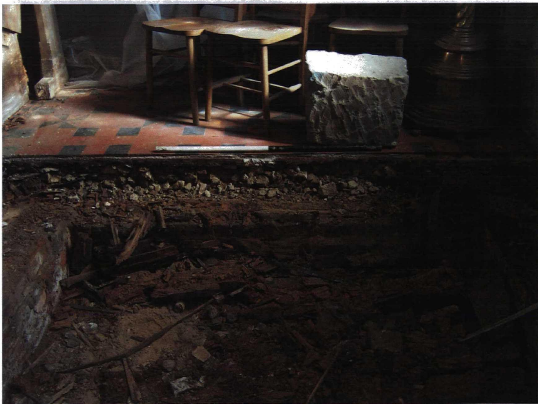
Plate 16 19 th century floor (2001) and associated hardcore overlying 19 th century brick foundations (2004), at the eastern end of the southern pews, viewed from the west.
