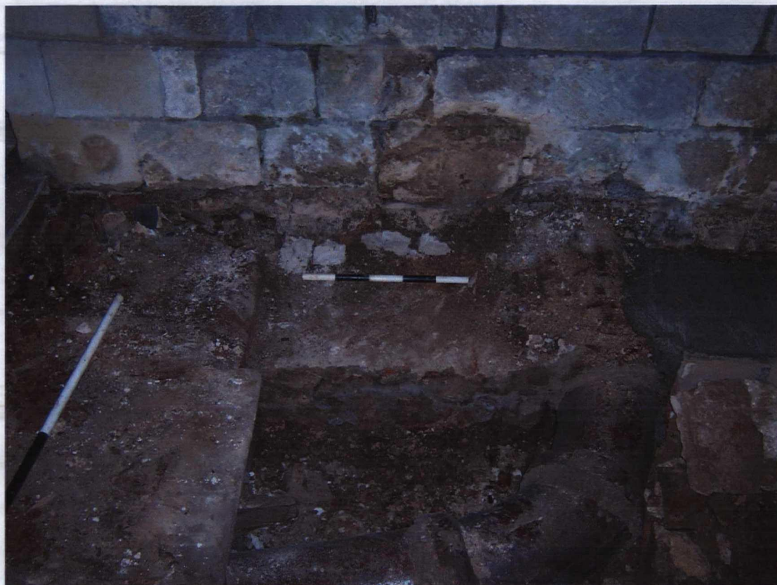
Plate 5 Brick underpinning (1020) for church wall (1021) overlying compact chalky clays (1018), showing 19 th century air duct (1015) to right and mid left. Viewed from the south.
