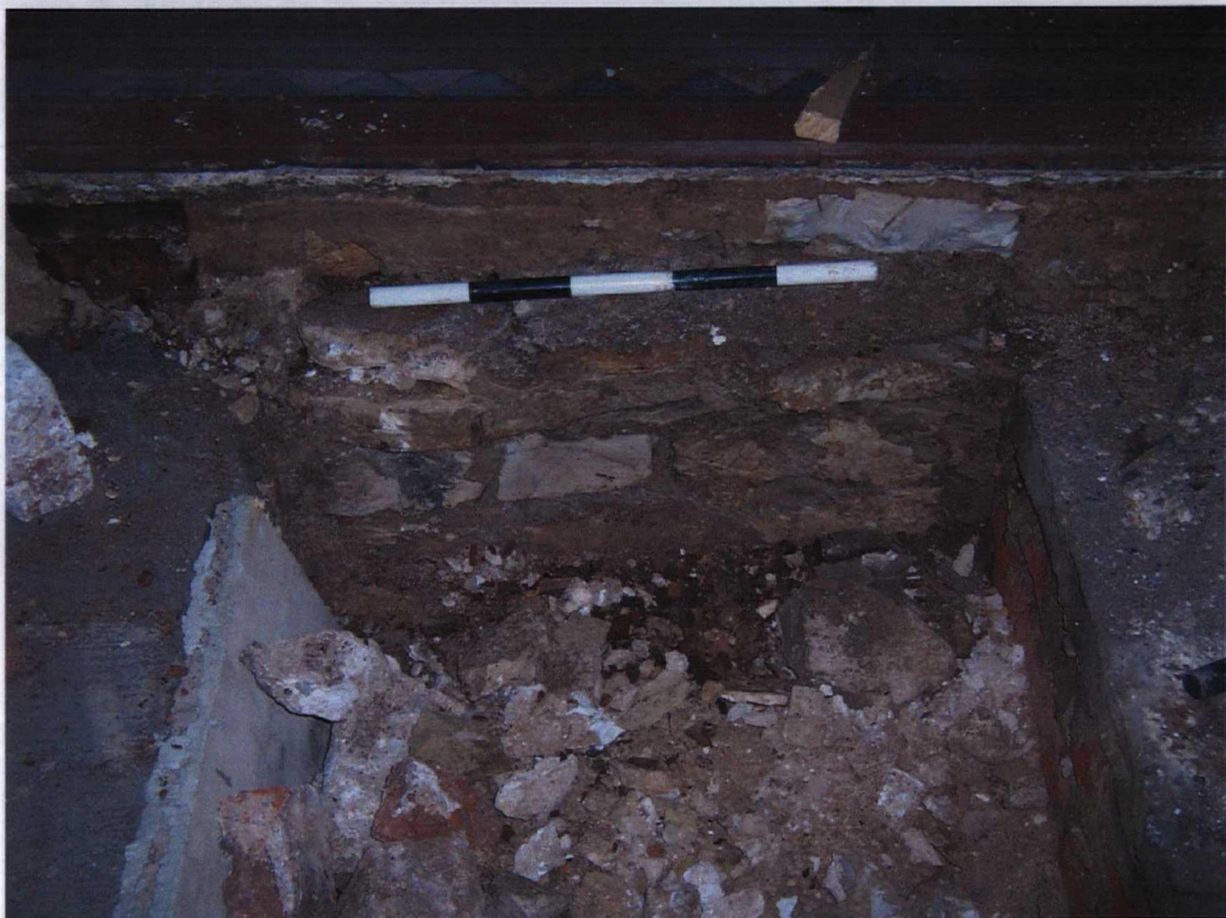
Plate 4 The isolated limestone foundations (1012), with concrete(1005) to the left and 19 th century brick services to the right, looking west.
