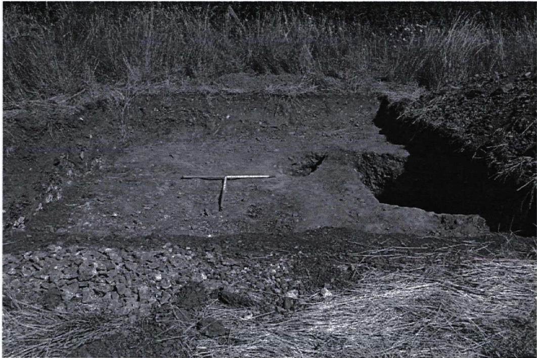
Plate 11. Trench 3. Post-Excavation. Facing East
