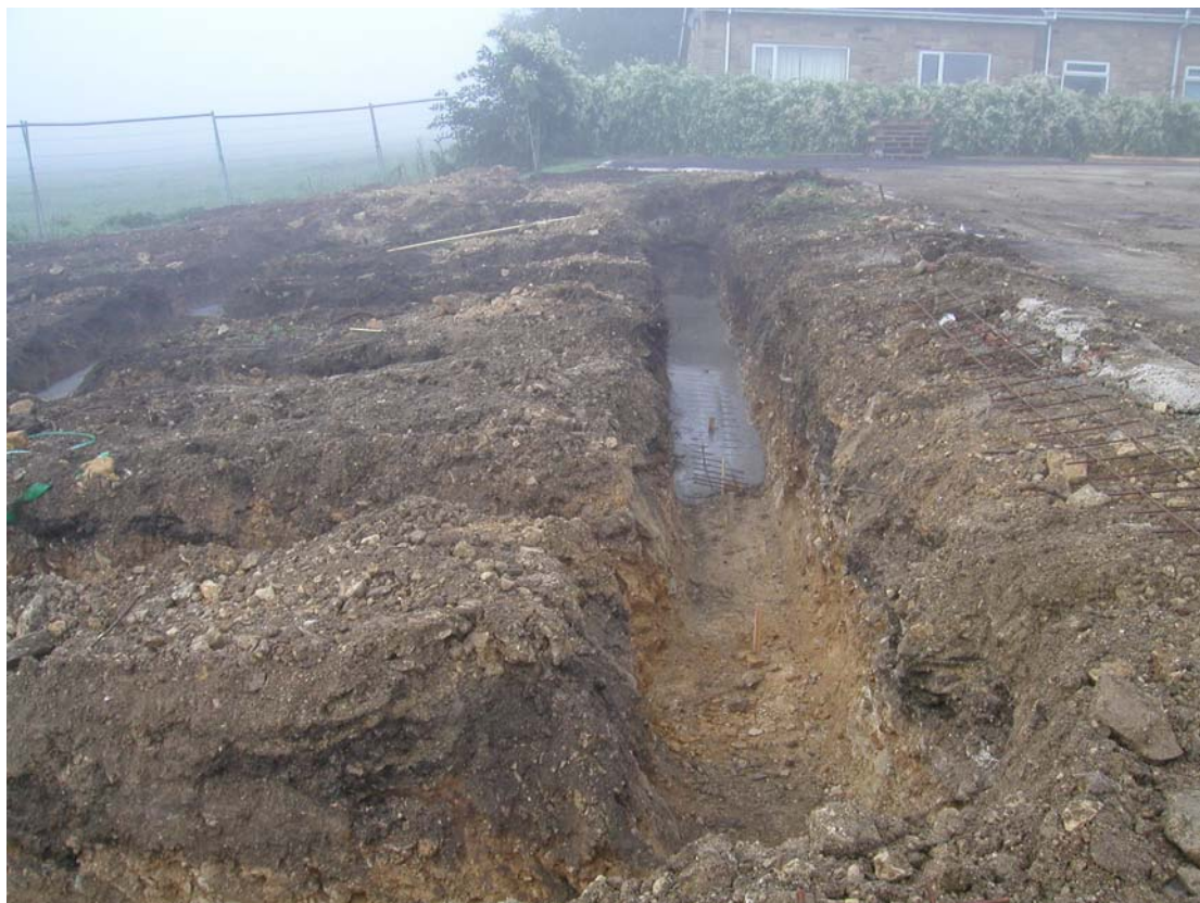
Plate 9 The foundations for plots 8 and 9
