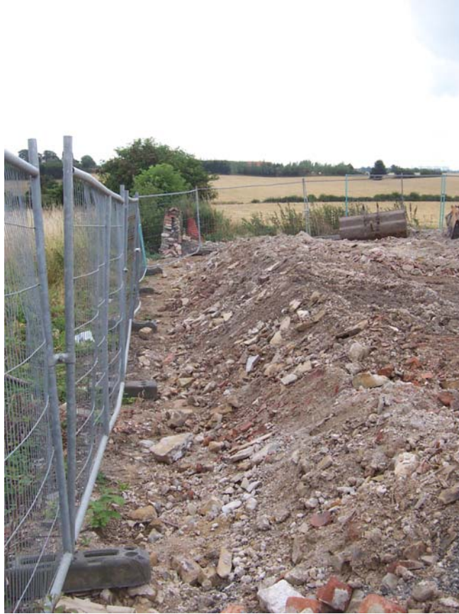
Plate 5 The southeast corner of the site during ground raising
