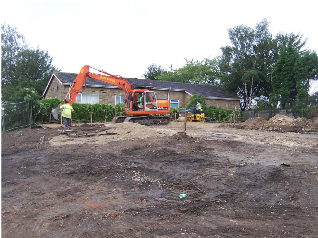
Plate 6 The access road under construction
