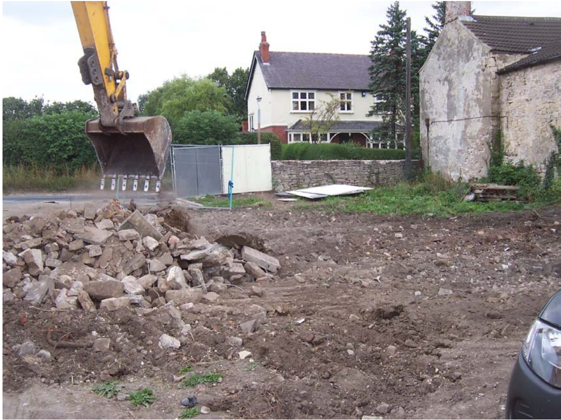
Plate 3 Demolition work in progress
