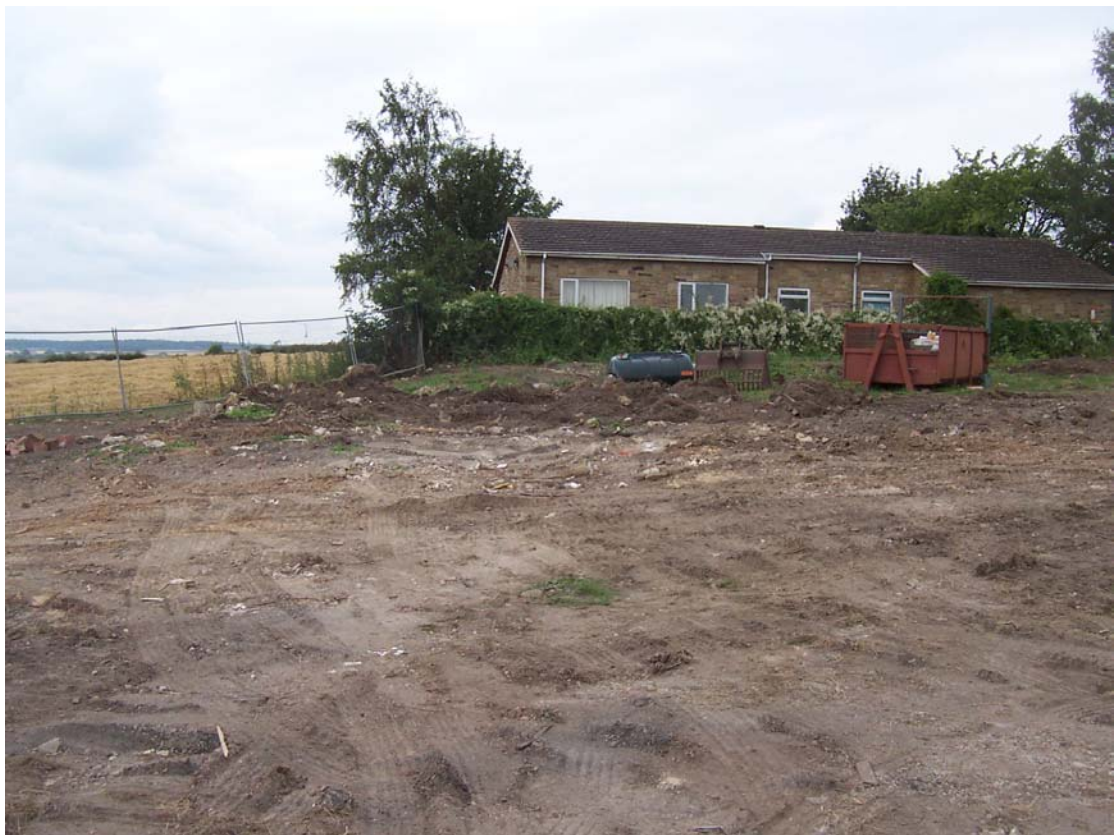
Plate 4 The west side of the site during clearance work
