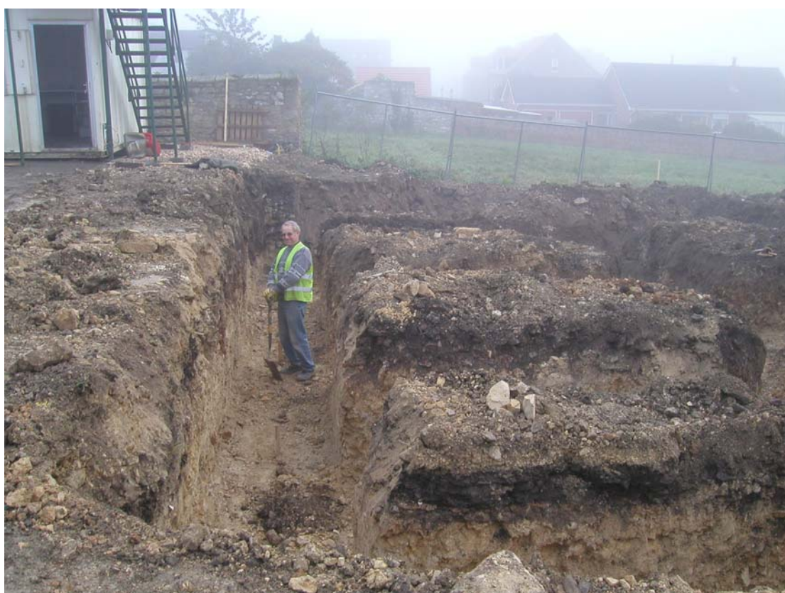
Plate 10 The foundations for plots 10 and 11
