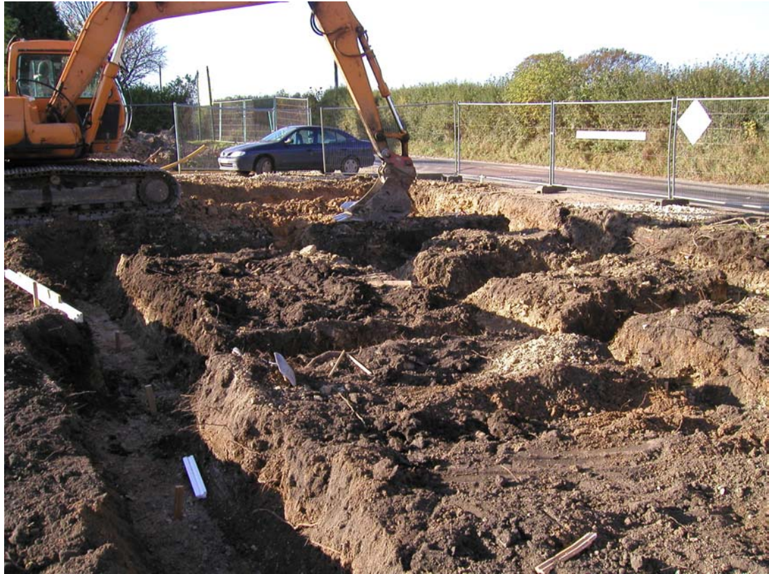
Plate 11 The foundations for plots 1 to 3
