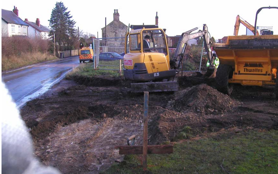
Plate 12 Work in progress on the new entrance
