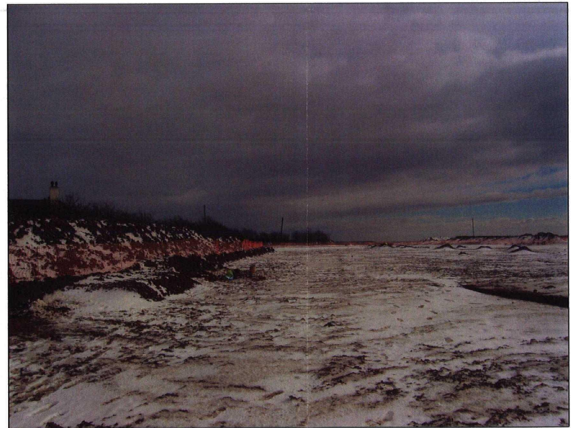
Plate 20. Working shot, after a snow storm looking southeast (Area B)
