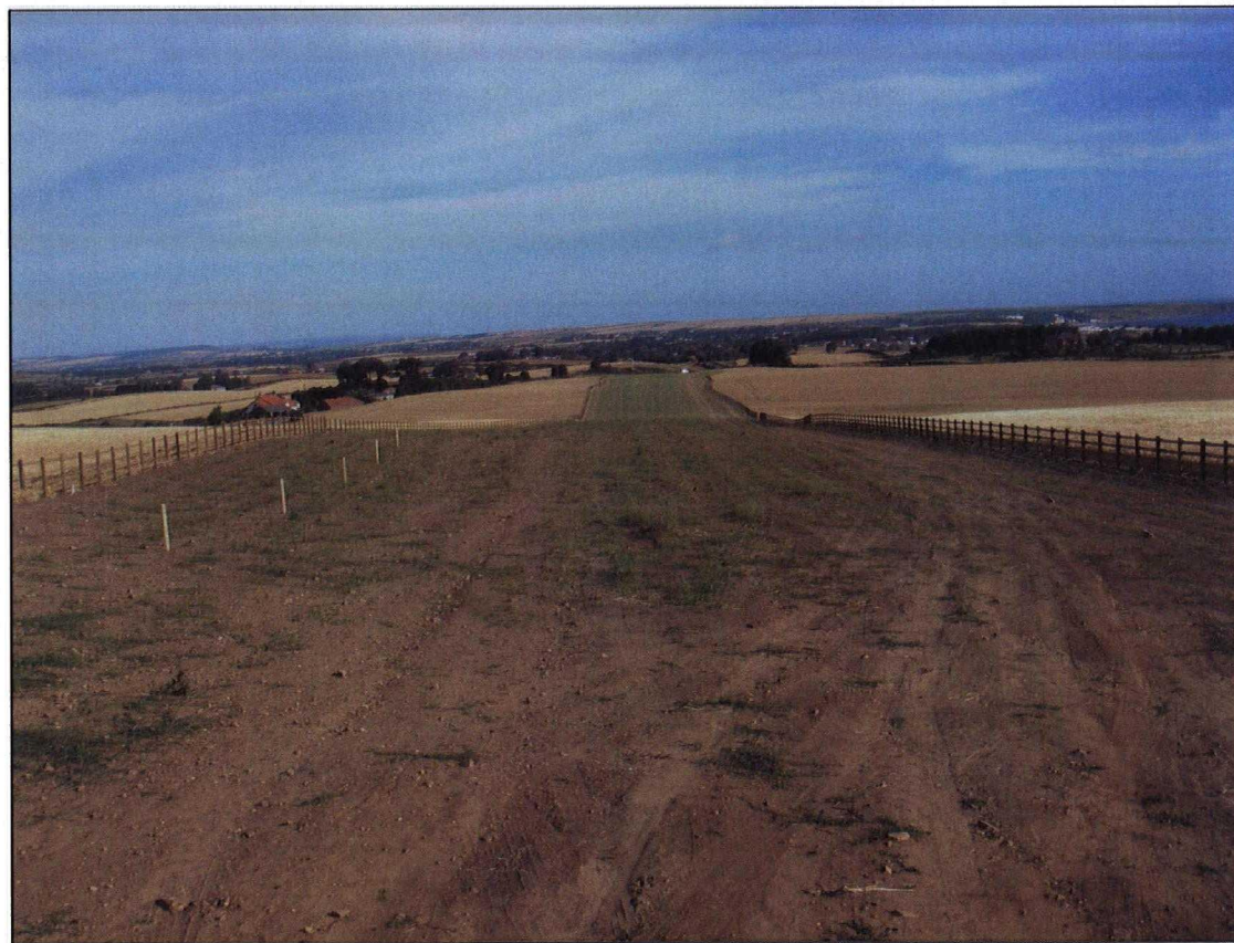
Plate 19. Stretch of the proposed A165 Bypass looking northwest (Areas F2, F3)
