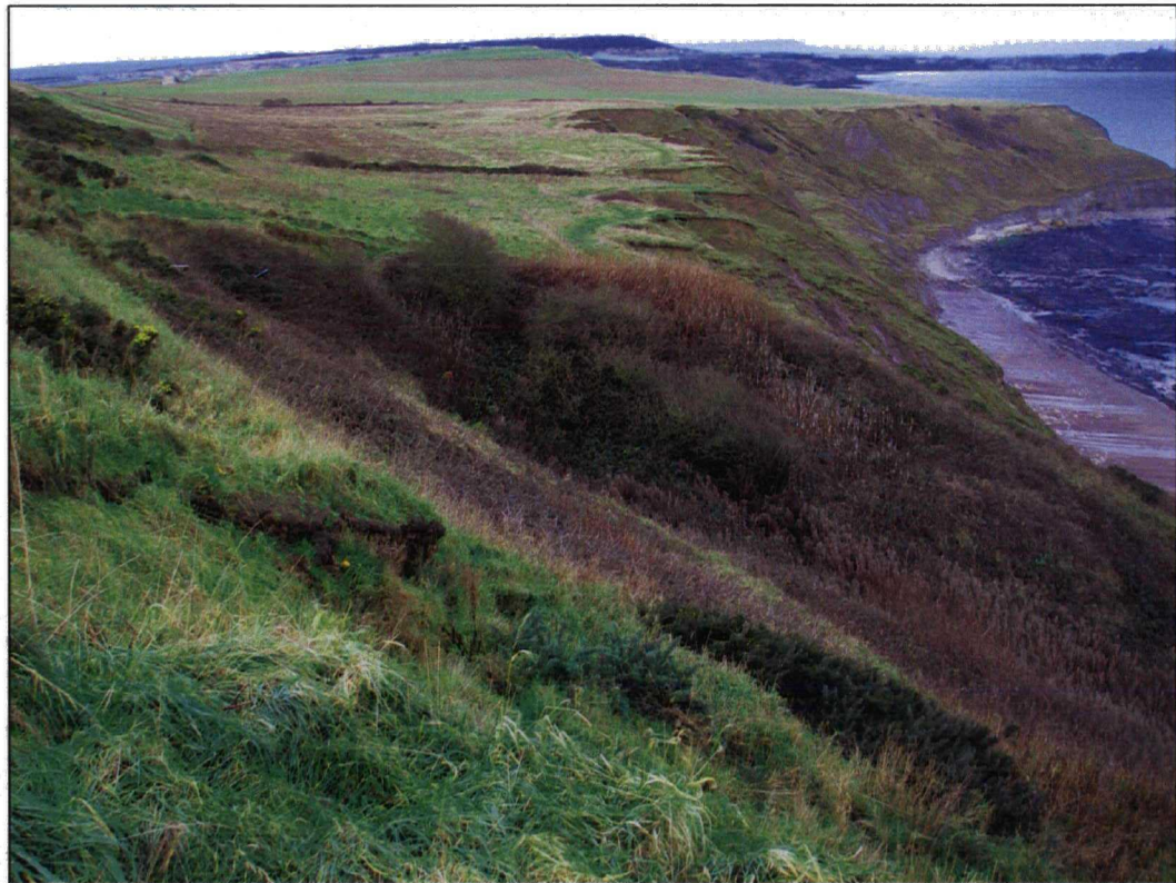
Plate 4. Site of a former sandstone quarry, on the cliff side to the north of the proposed redevelopment area
