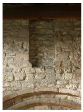
Fig. 17: Blocked doorway at first floor level in tower, seen from the nave
