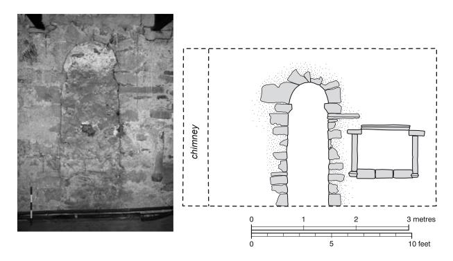
Fig. 16: Photograph and drawn elevation of blocked doorway in east wall of tower, and adjacent recess, showing inter alia the extent of mortar/plaster rendering
