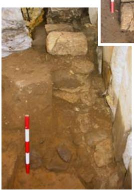
Fig. 23a (below): Southern aisle wall structure and foundation seen in section; Fig.23b (inset) two oolitic limestone blocks, one interposed below on overhanging stone in the tower wall, viewed from above. Scale unit: 100 mm.
