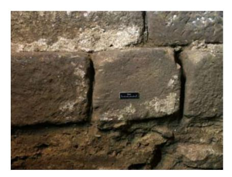
Fig. 10: Plaster/ render on internal face of reused gritstone blocks in the foundation for the tower's west wall.
