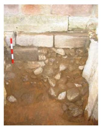
Fig. 11: The junction between gritstone block and rubble foundations for the standing tower, over the earlier cobble foundations, below the south wall of the tower. Scale unit 100 mm.
