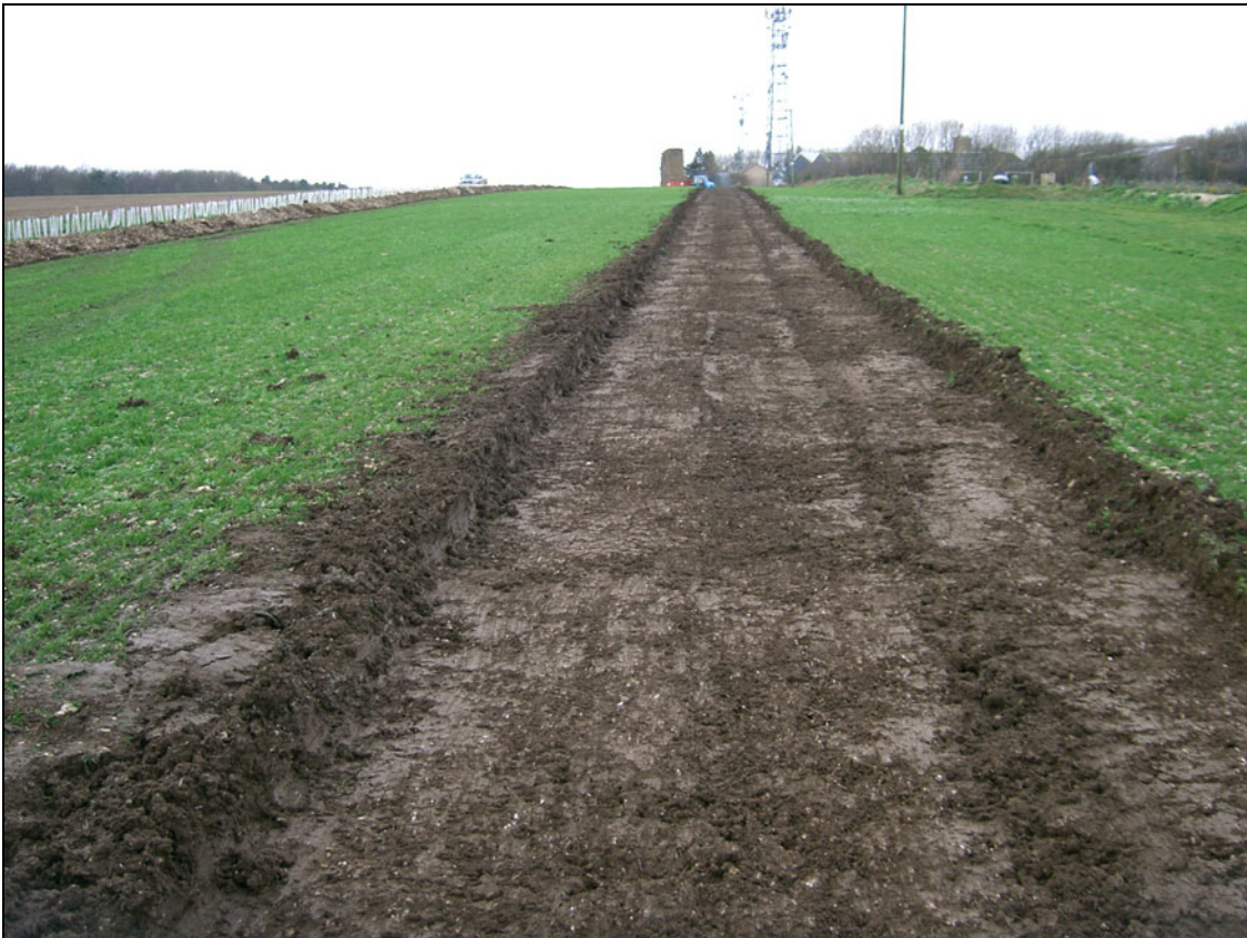
Figure 7 The road trench looking west towards West Farm.
