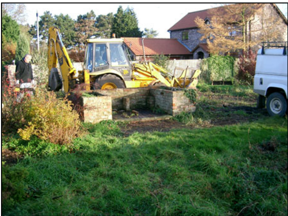
Figure 3 Brick-built raised flower bed
