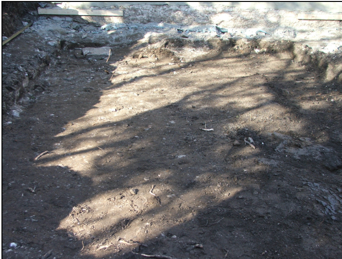
Figure 5 The foundation area, looking north, prior to the excavation of the wall trenches. The uppermost slab of culvert [18] can be seen at the top left of the frame
