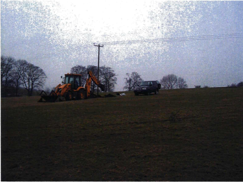
Plate 1. General View of Site. Facing North West
