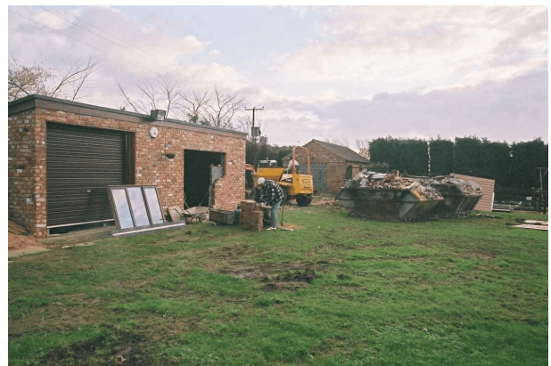
Plate 1 General site view
