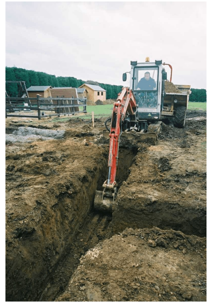
Plate 3 Machining trenches
