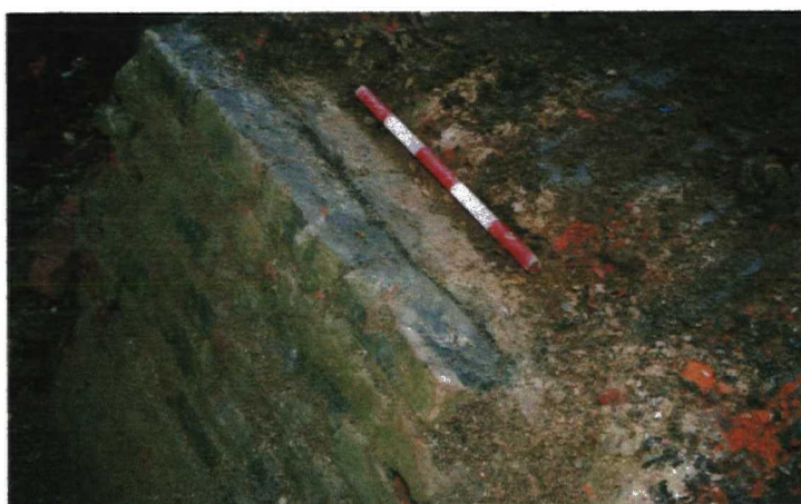
Figure 1 Film 1 frame 5 showing the wall thought to be a barrel drop for the basement to the former works building Scale 500mm
