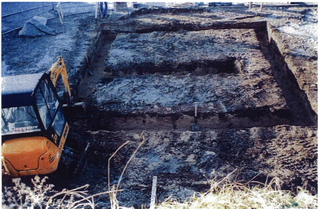
Plate 2. Excavated Foundations for House Plot. Facing West
