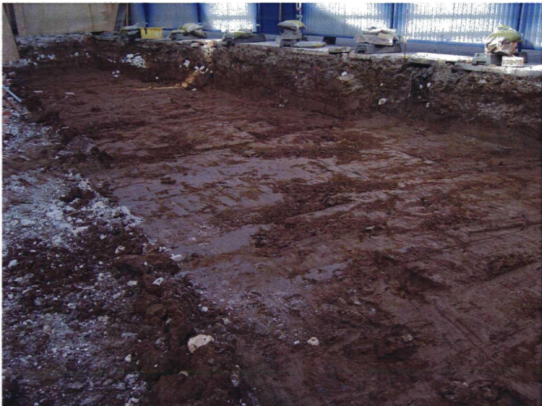
Plate 2. Southern Area of Site after Stripping. Facing South West
