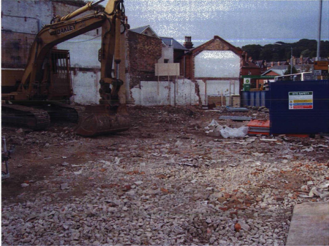
Plate 1. General View of Site. Facing South West
