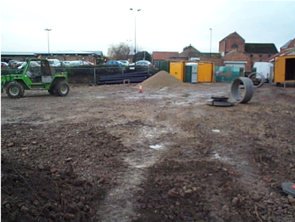
Plate 1. General View of Site. Facing South West
