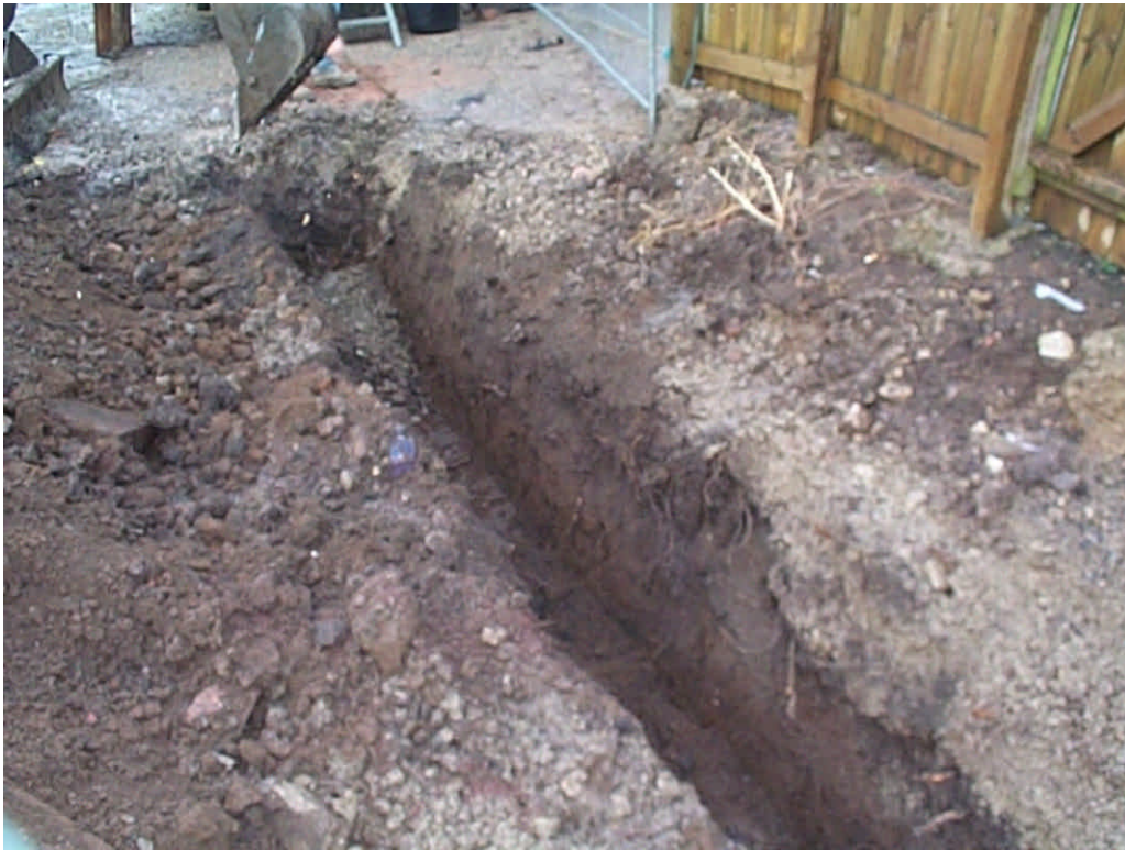
Plate 3. View of Drain Trench. Facing North West
