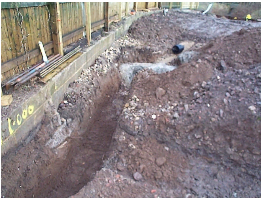
Plate 2. View of Drain Trench. Facing East
