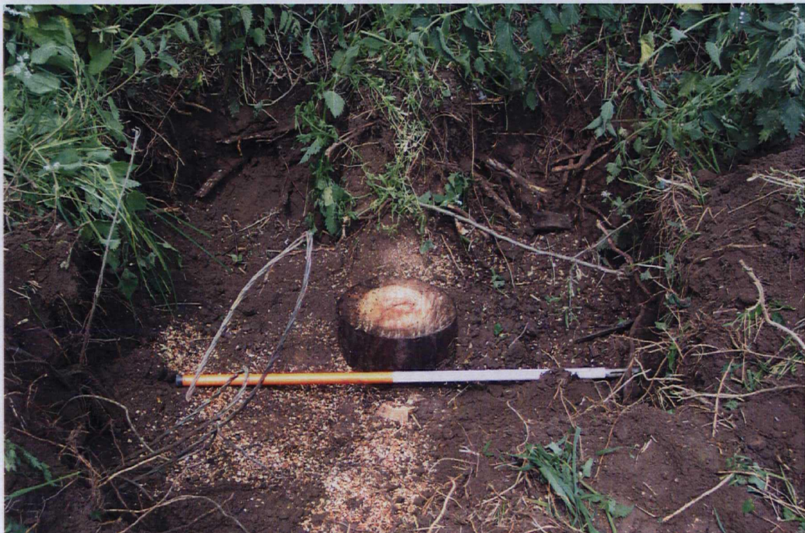
Plate 4. Pole 1. Completed Excavations. Facing North
