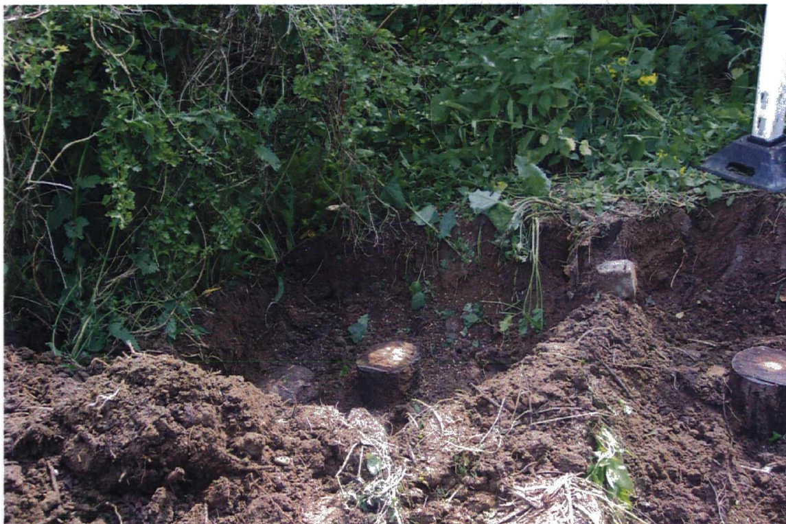
Plate 6. Poles 2 & 3. Completed Excavations. Facing South
