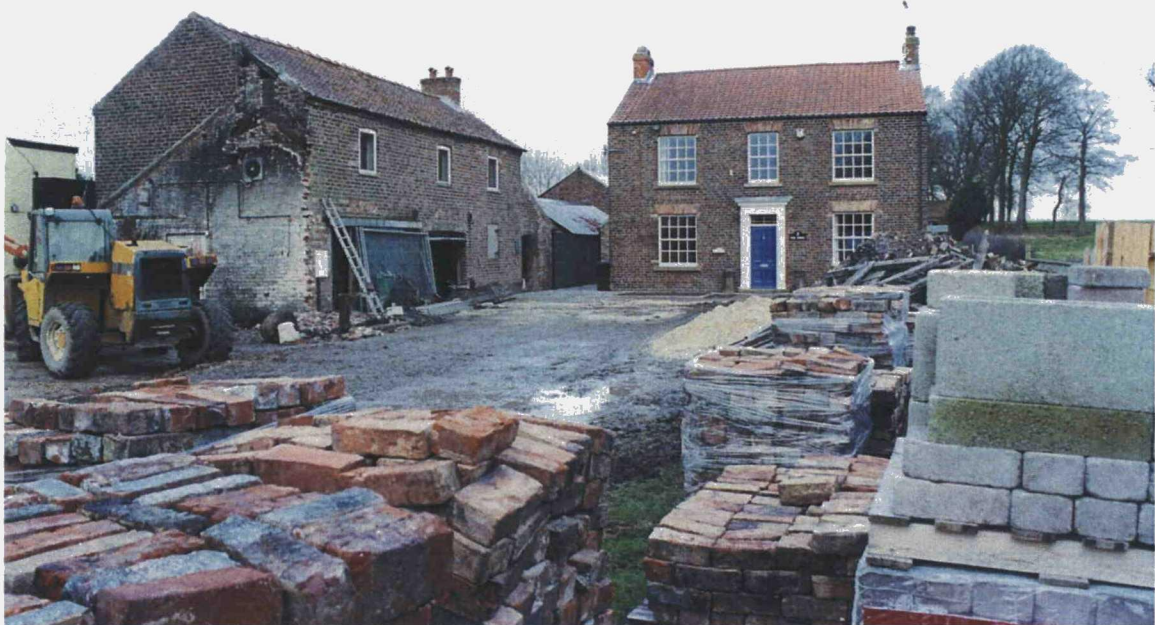
Plate 2. General View of Site. Facing North West
