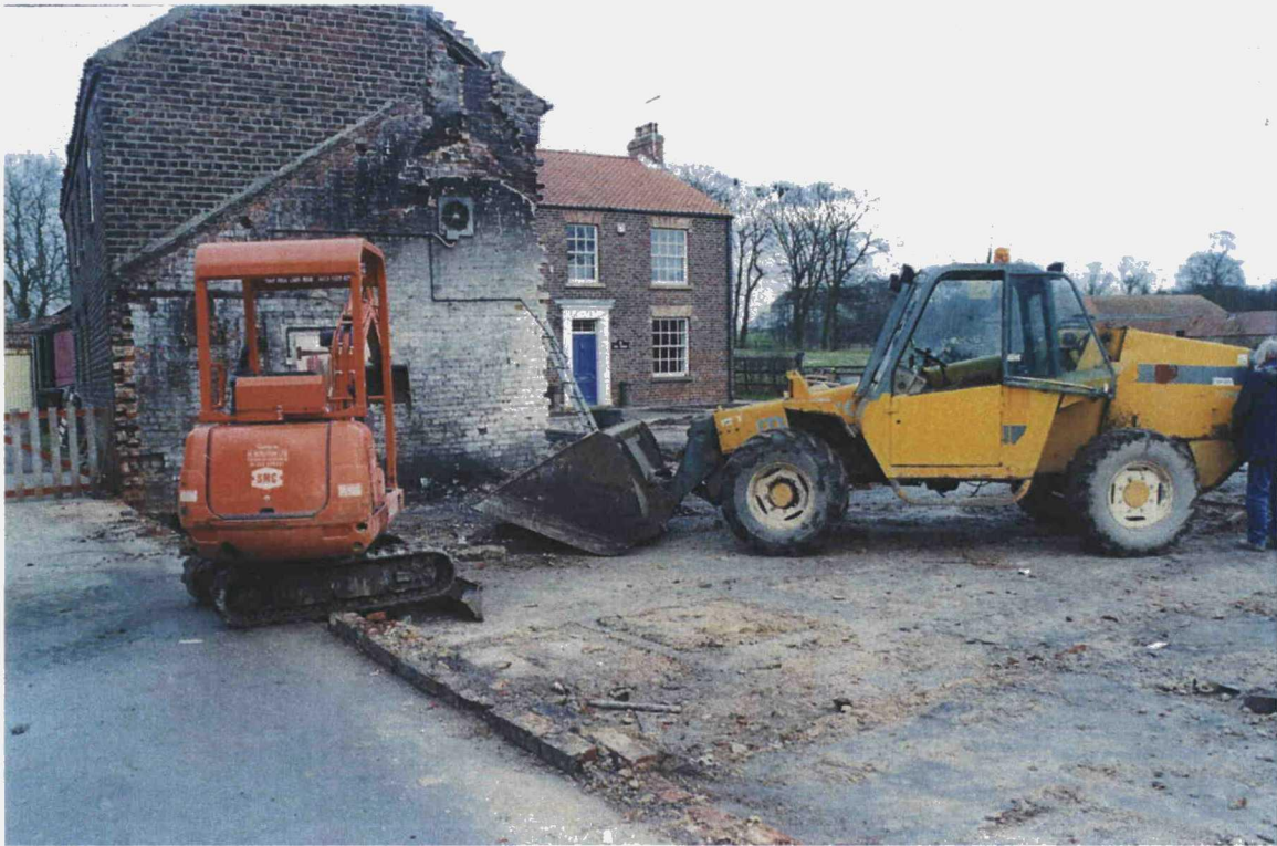
Plate 1. General View of Site. Facing North East
