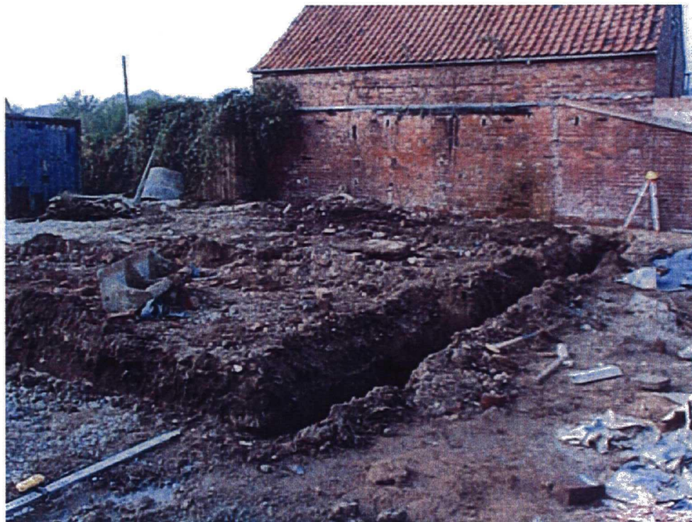
Plate 8. Overall View of Foundations. Facing North West
