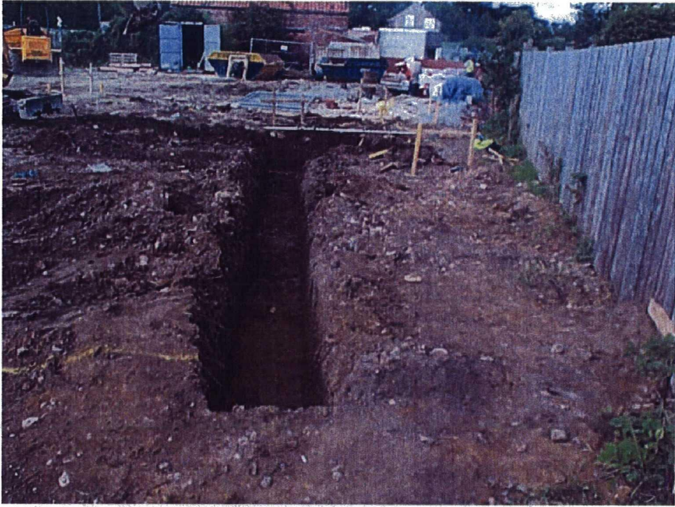
Plate 5. South East Foundation Unit 7. Facing North
