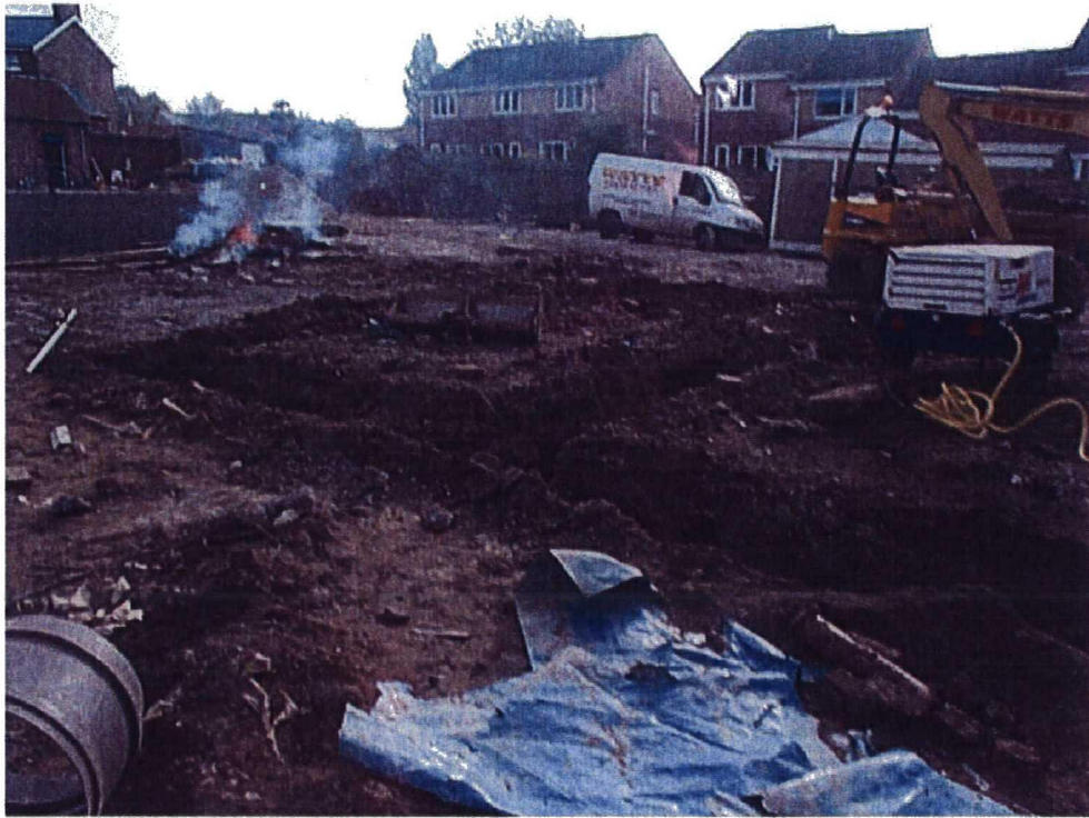
Plate 9. Overall View of Foundations. Facing West
