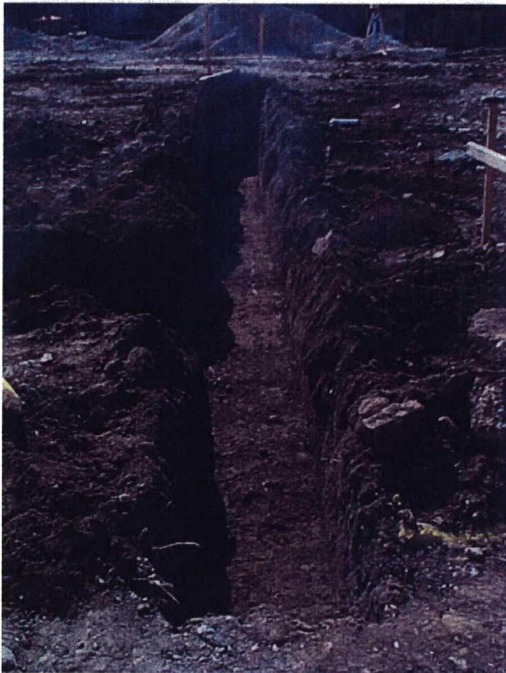
Plate 6. Northern Foundation Unit 7. Facing West
