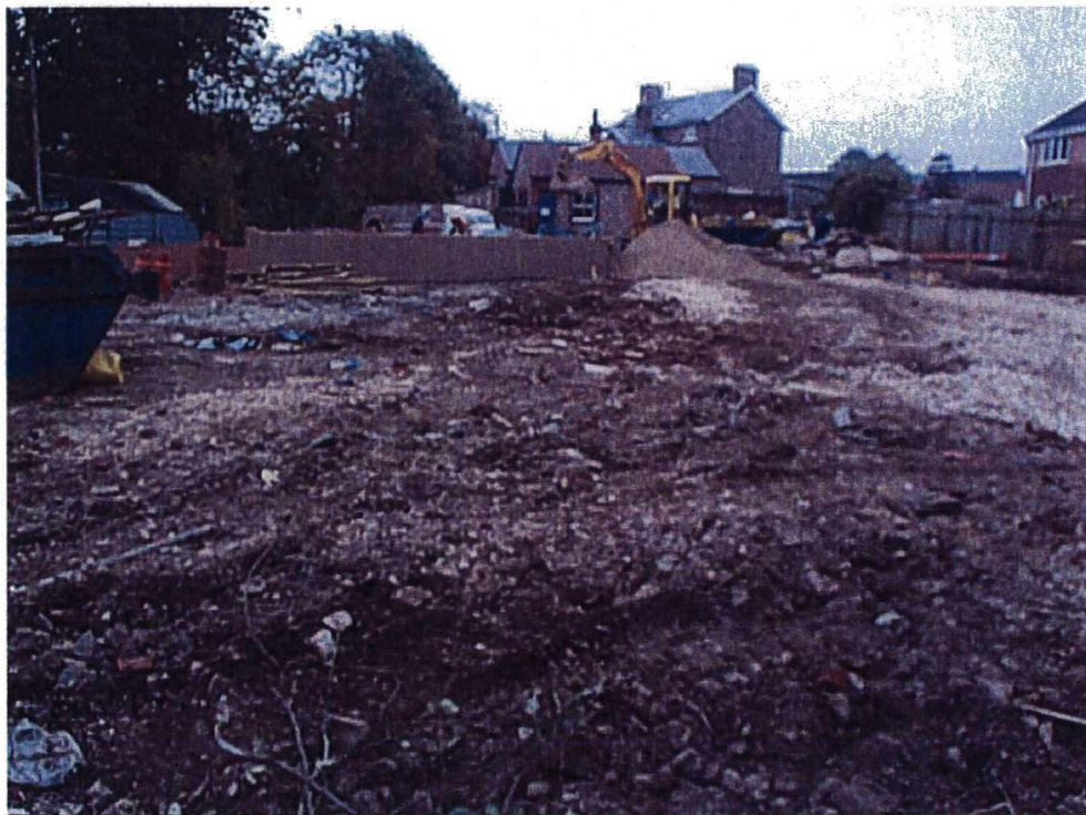
Plate 2. General View of Site. Facing South West
