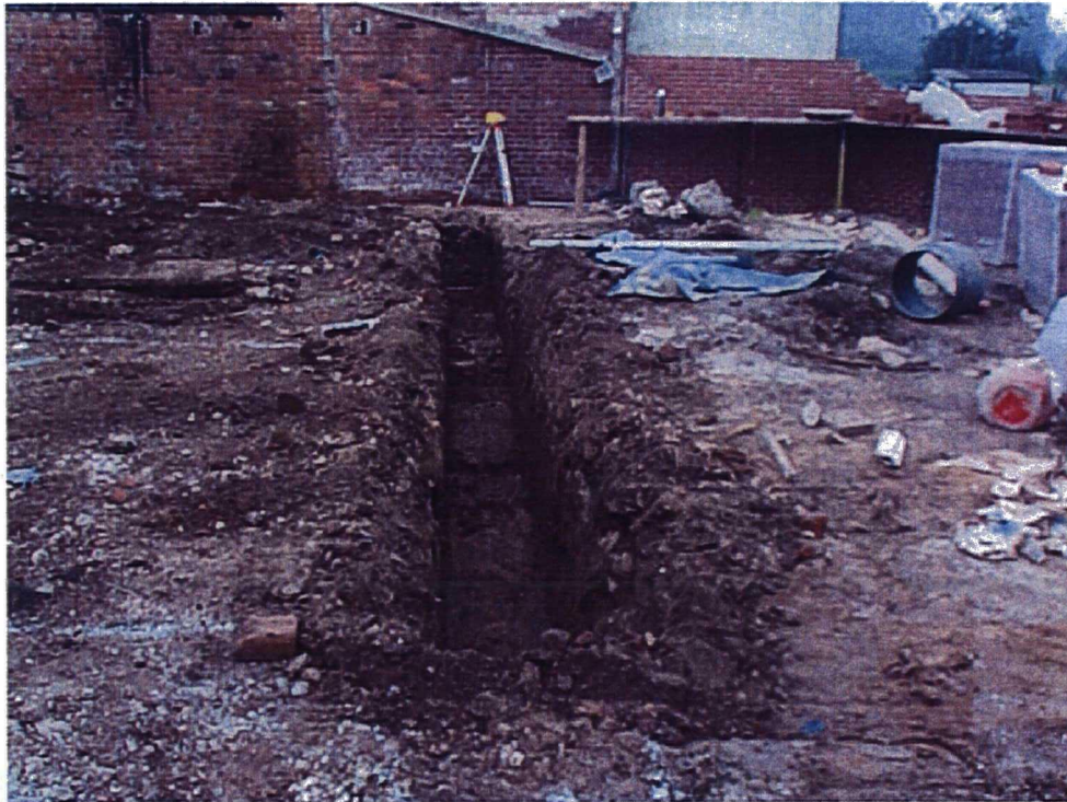
Plate 7. Excavation of Eastern Foundation Units 1-3. Facing North
